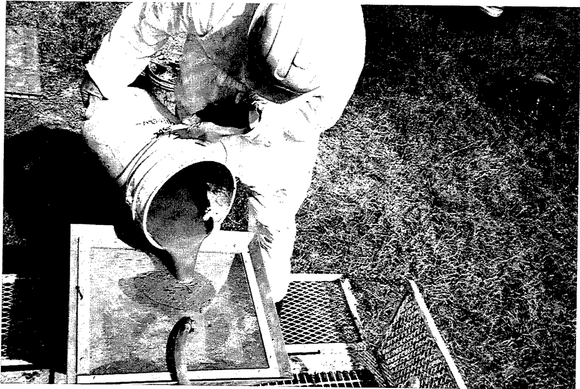
Figure 6. Pouring grout mix through the hopper screen
