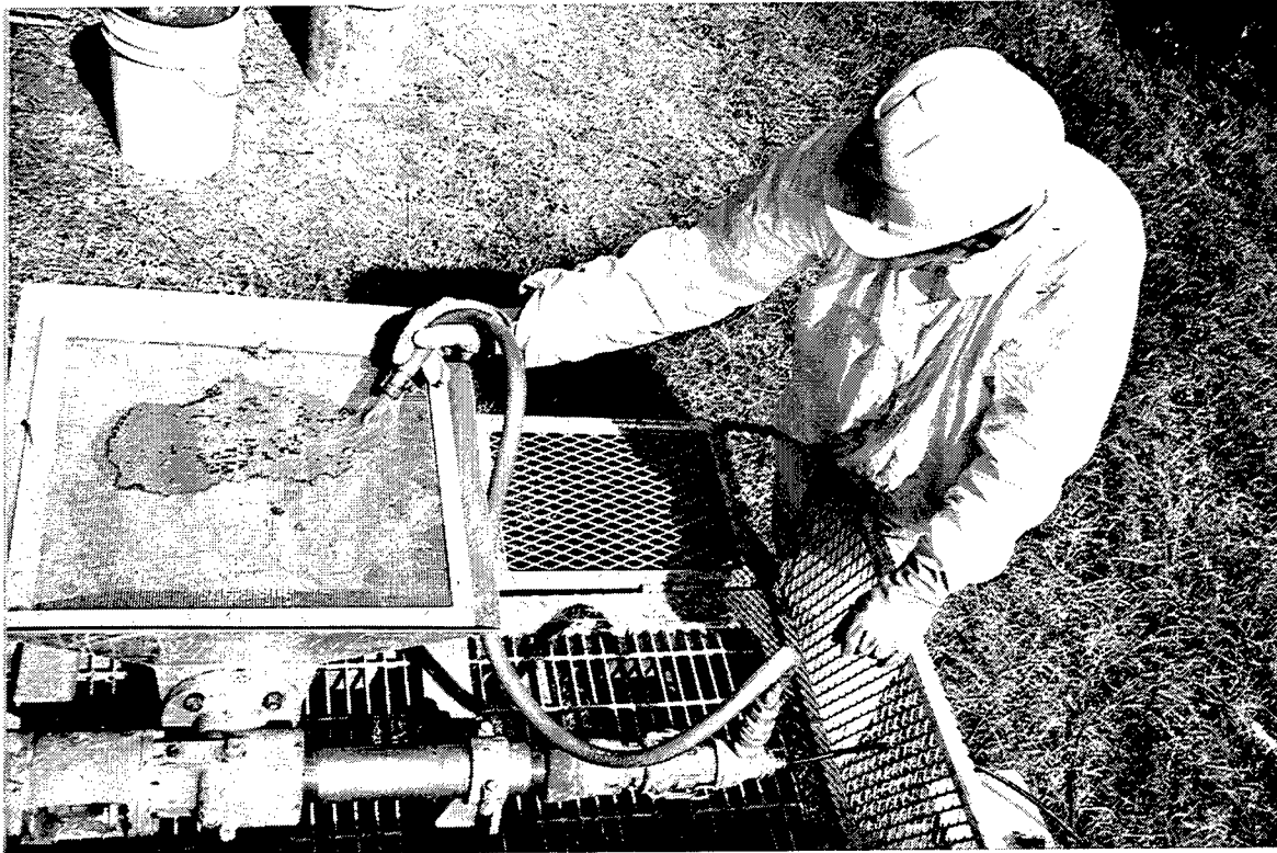
Figure 7. Recirculating grout into the hopper
