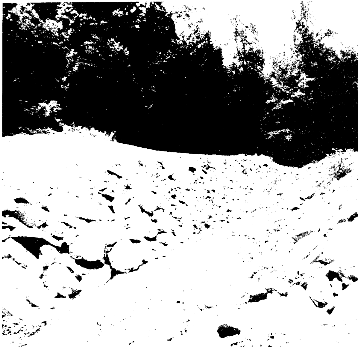
Figure 3.3-13. Use of riprap to protect a streambank from erosion (from U.S. Environmental Protection Agency 1976).
