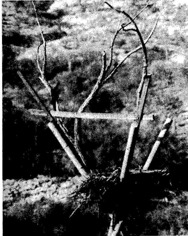
Figure 3.3-23. Finished tripod apex with attachments (from Grubb 1980).
