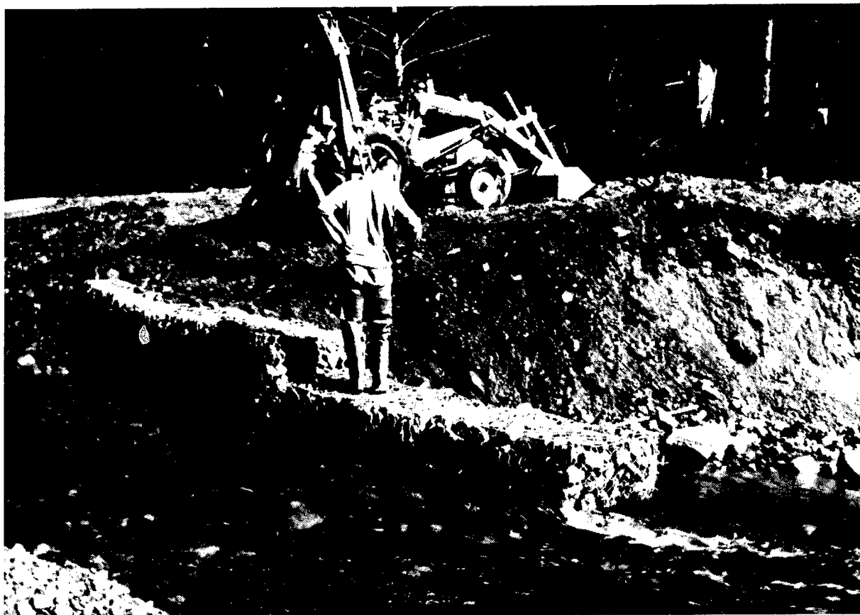
Figure 3.3-11. Placement of stone gabion to protect a streambank (from U.S. Forest Service 1969).
