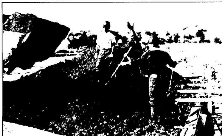
Figure 1. Preparing contaminated soil piles for biopile remediation.
