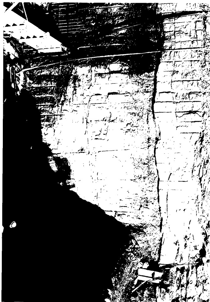
(155) L-5 View of East Wall
