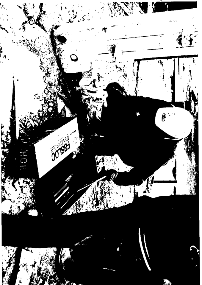
(208) Inserting Fastloc Resin (210) Inserting Rods into Hole
