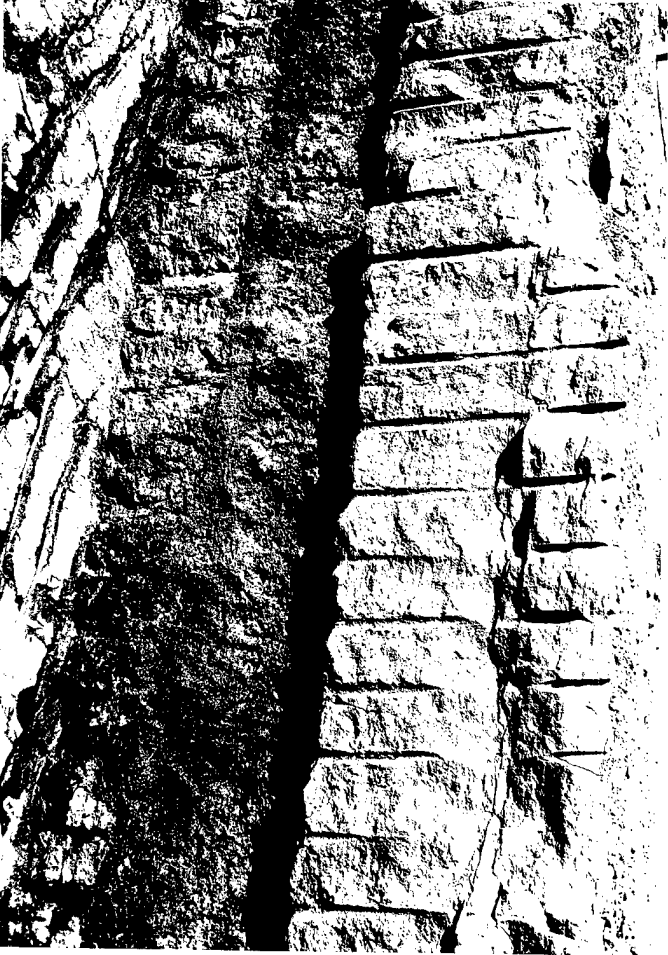
(193) RC-16 View of Western wall
