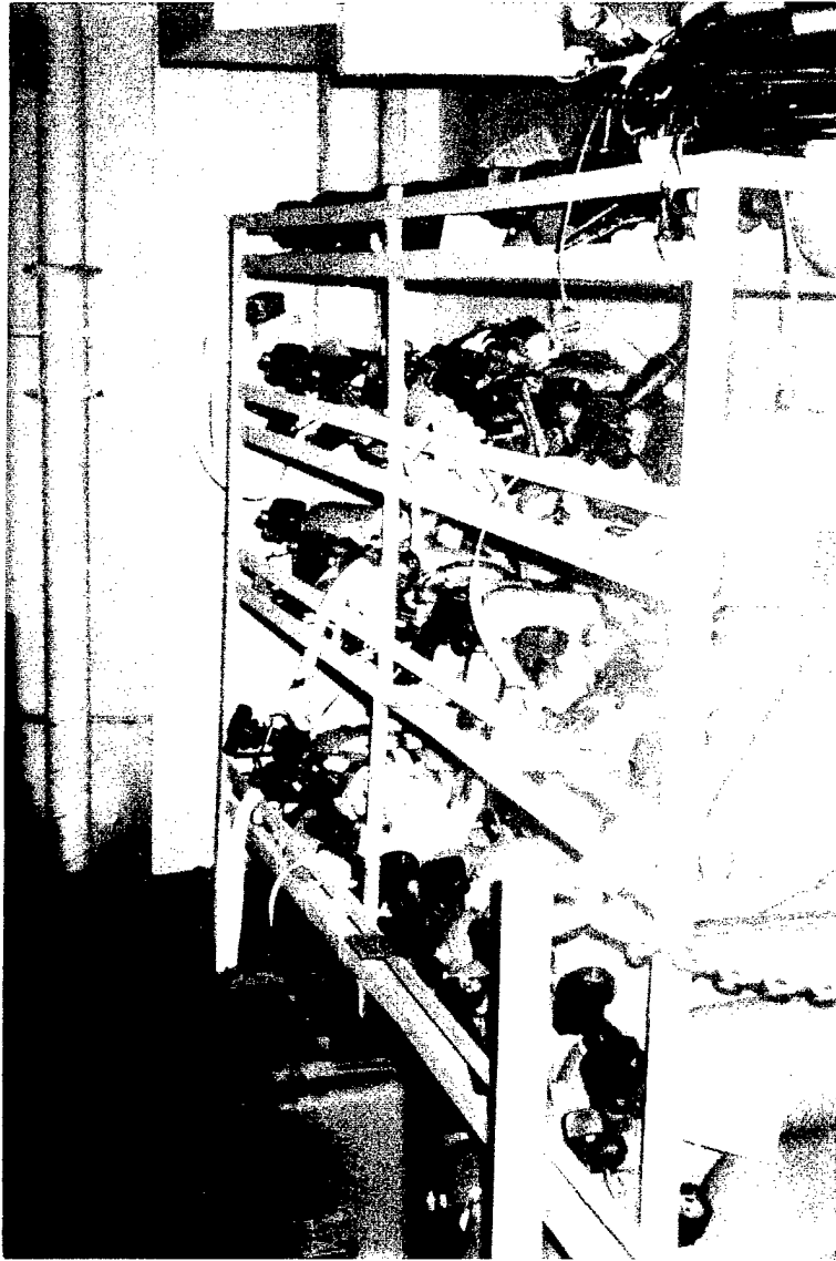
Fig. 17 — SCBA Storage in former Paint Locker (2-0-2-A)
