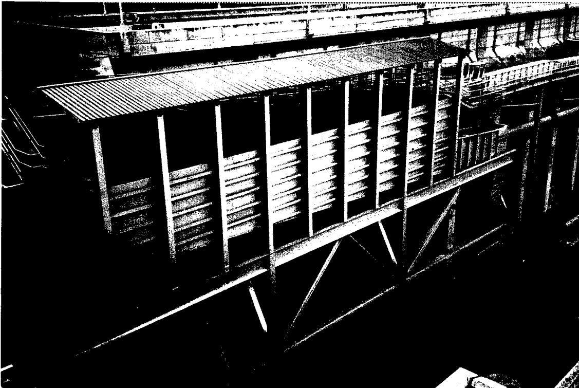
Dewatering facility (flow from left to right) discharging into corrugated metal flume (CMF) with shade cover.
