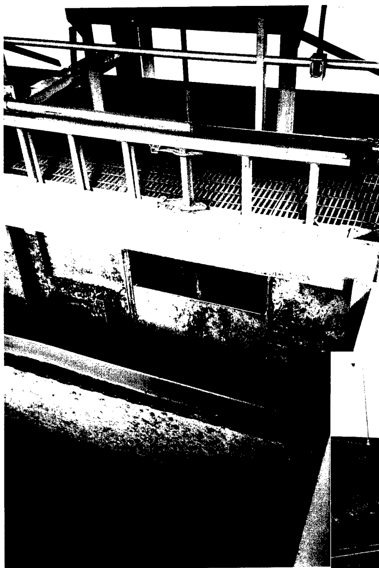
One of six weir gates to control floor dewatering discharge.
