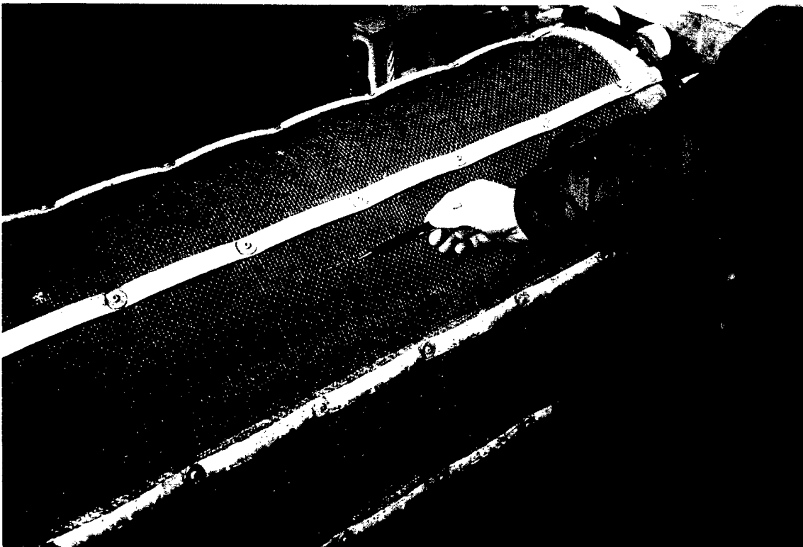
Close-up view of plastic mesh screen used in STS's. (Similar at all projects visited.)
