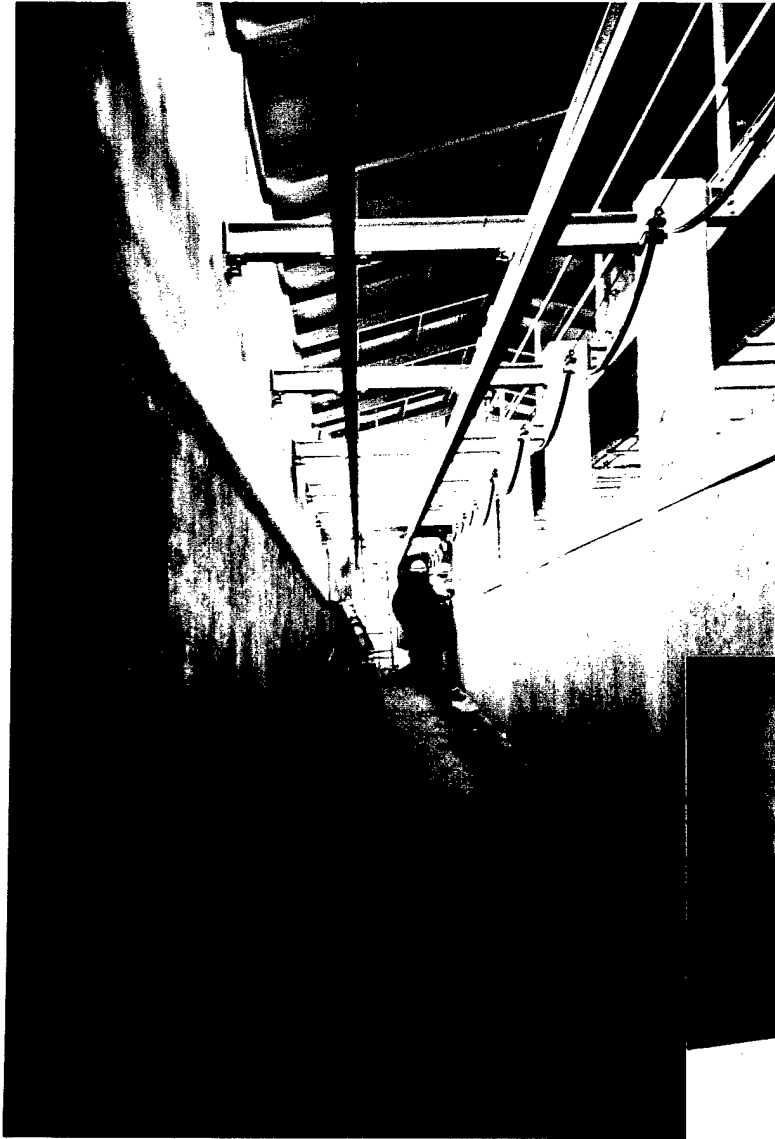
Dewatering facility with emergency overflow weirs along right wall. Floor screens covered with plywood during maintenance work.
