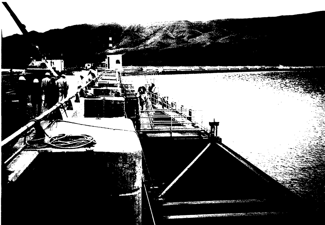
Downstream view of the collection/dewatering system with stainless steel perforated plate in converging walls beneath walkways. Coarse trashrack in lower center of photo. Control panels for blower pumps beyond
