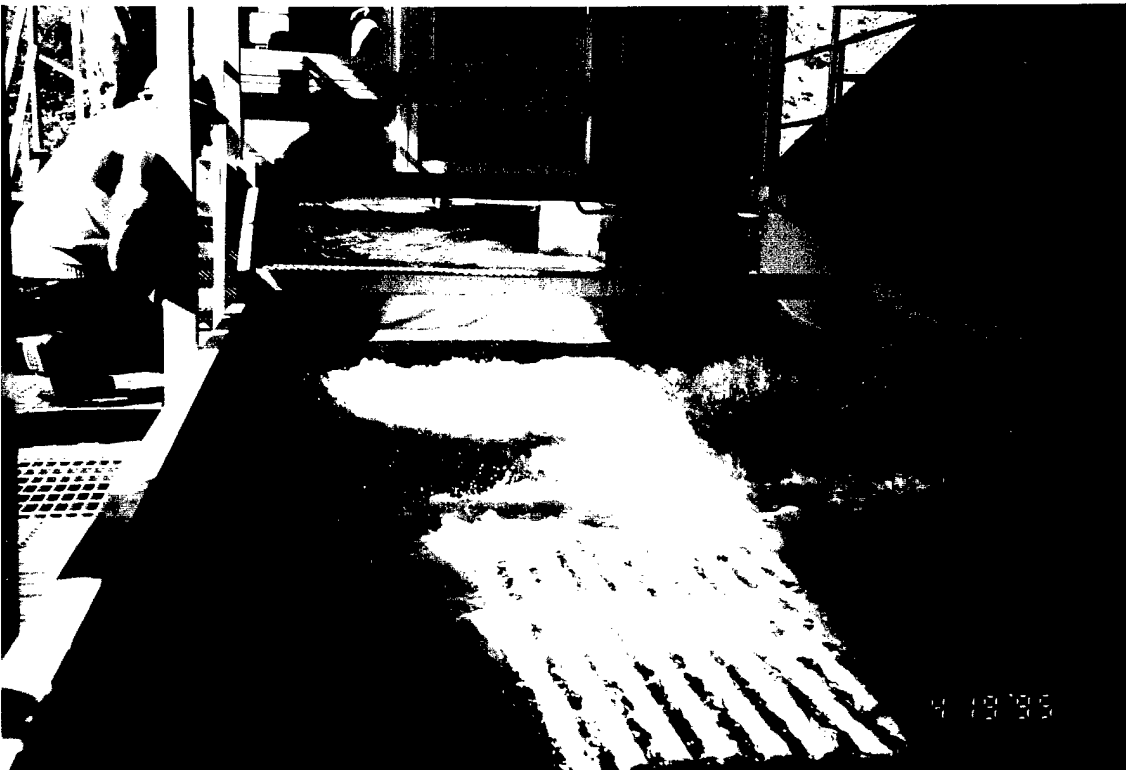
Upstream view of bypass discharge from upwell, passing through primary and secondary dewatering systems, and entering fish separator in lower portion of photo.
