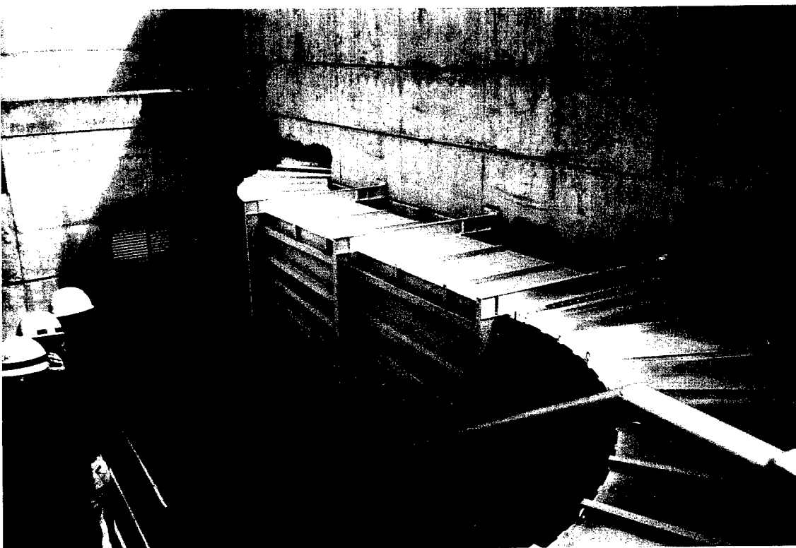
Fish collection flume exiting dam extending to dewatering facilities.
