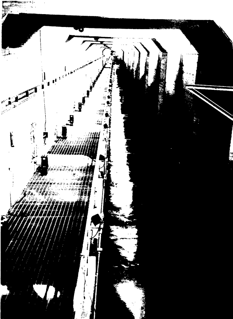
Ice/trash sluiceway converted to juvenile fish collection channel looking upstream. Knife gate operators for gatewell orifices above grating along left wall.
