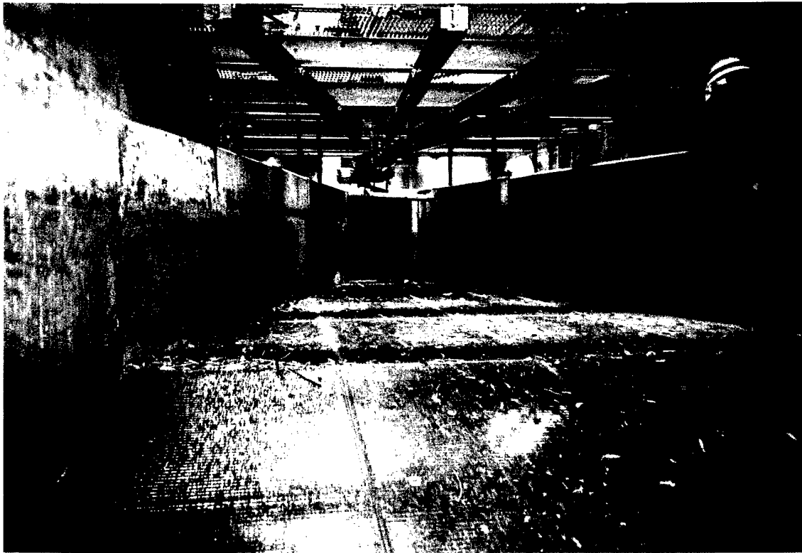
Floor dewatering system with bar screens looking downstream with converging walls and inclined floor screens. Beams mounted above support brush cleaning systems in converging section.
