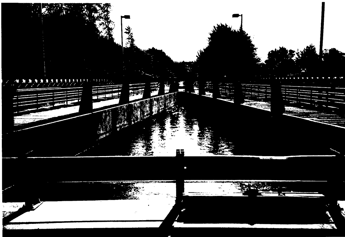
Downstream view of converging screening facility with vertical screens and adjustable porosity vanes. Bypass piping with weir gate at downstream end of converging section. Screen cleaning system rails along converging section deck.
