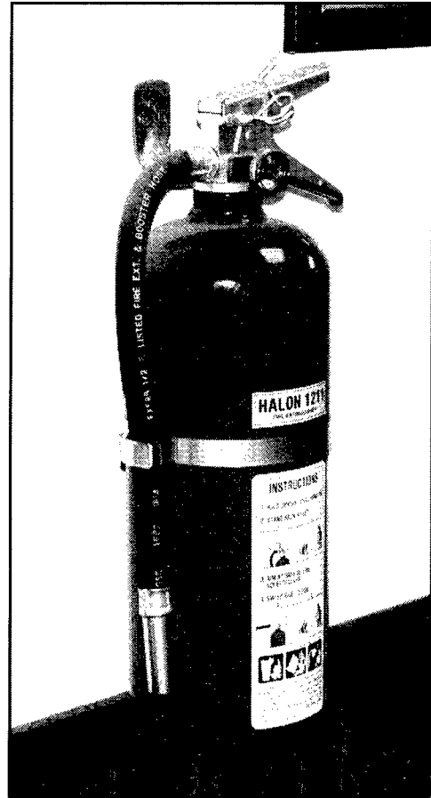
Figure 3. Halon fire extinguisher in Building 661.
