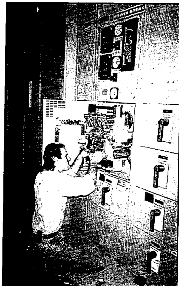
Main switch gear undergoing emergency repair
