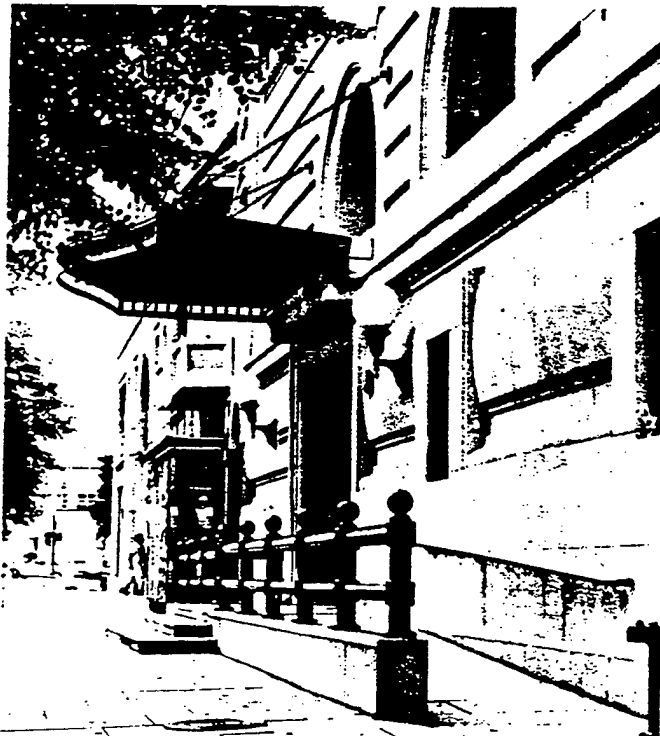
Figure 9. This ramp was created by infilling the window-well and slightly modifying the historic railing. The ramp preserves this building's historic character. Photo: Thomas Jester.
