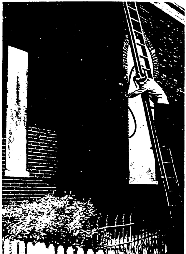
"Line Drop." Even though the operator of the sandblasting equipment is standing on a ladder to reach the higher sections of the wall, it is still almost impossible to have total control over the pressure. The pressure of the sand hitting the lower portion of the wall will still be greater than that above, because of the "line drop" in the distance from the pressure source to the nozzle. (Hugh Miller)
