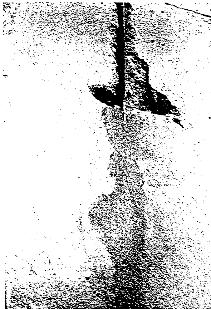
Fig. 12. Without proper preparation and correction of a pre-existing problem, repairs will fail. Insufficient concrete at the surface caused this patch around a reinforcing bar to fail within a year. In this case, a structural engineer should have assessed the need for this rod so close to the surface. Redundant rods are often cut out prior to patching. Photo: Alonzo White.
