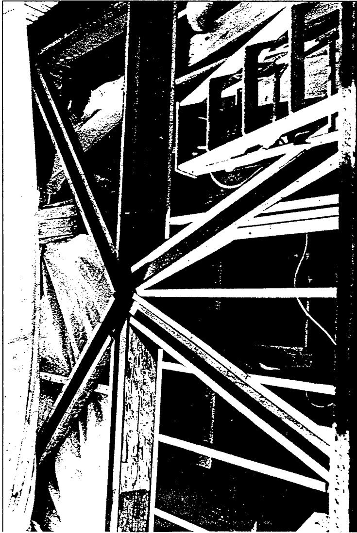
In order to preserve this historic wood-frame building, new steel framing was inserted to reinforce the wood post and beam structure. Original wood framing members were notched to accommodate the new steel frame.
