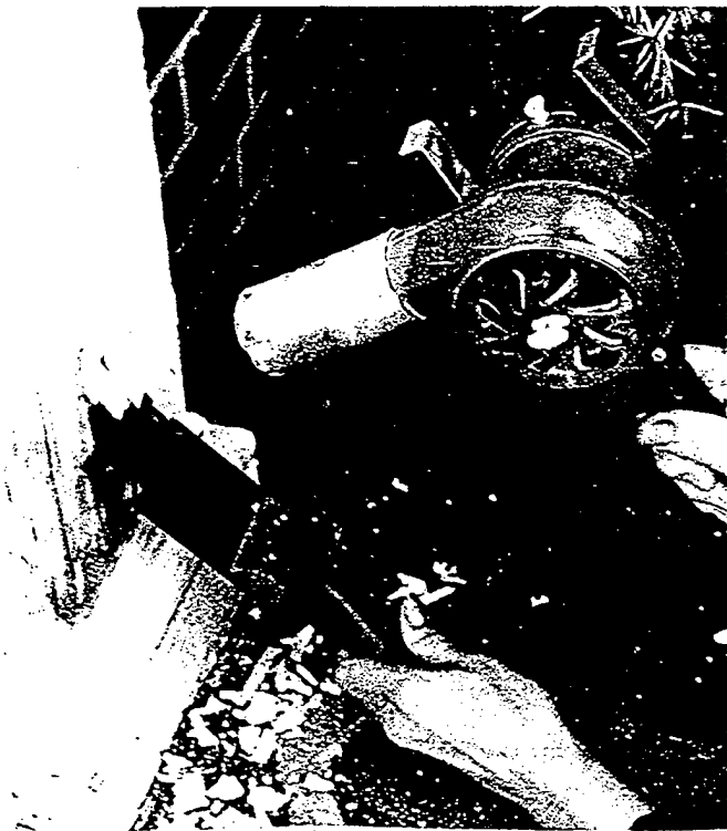
Fig. 14 The nozzle on the electric heat gun permits hot air to be aimed into cavities on solid decorative elements such as this applied column. After the paint has been sufficiently softened, it can be removed with a profiled scraper. Photo: Charles E. Fisher, III.
