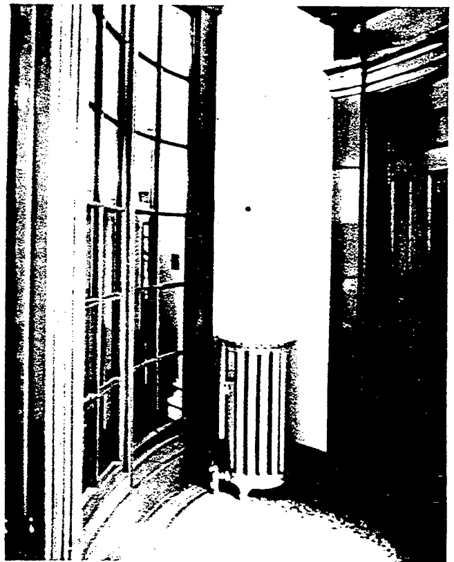
6. A condition assessment during the planning stage would identify this round radiator in a small oval-shaped vestibule as a significant element of the historic heating system. In upgrading the mechanical system, the radiator should be retained. Photo: Michael C. Henry, P.E., AIA.
