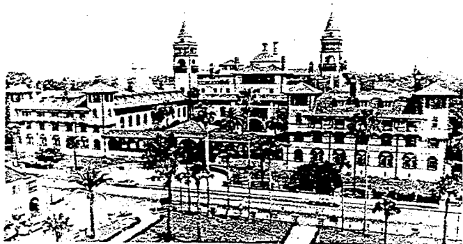
Fig. 3. Ponce de Leon Hotel, St. Augustine, Florida (1885-87). An example of unreinforced concrete used on a grand scale, this Spanish Colonial Revival hotel was designed by Carrere and Hastings and commissioned by railroad magnate Henry Flagler. The building now serves as the main campus hall for Flagler College. Photo: Flagler College.
