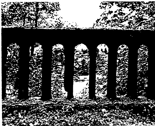
Fig. 15a. The spindle-type railings were deteriorated beyond repair. The concrete was cracked or broken and the center reinforcing rods were exposed and badly rusted.
