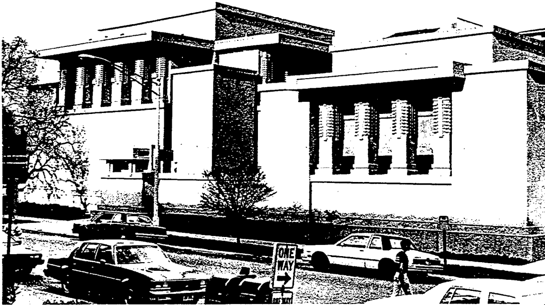
Fig. 14c. Once the repair work was complete, the entire building was sprayed with a concrete mixture consisting of pea-gravel, cement, and sand, which was then hand-
