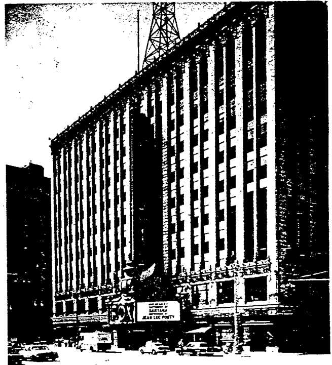
3. The circa 1928 Fox Theater in Detroit, designed by C. Howard Crane, was one of the earliest twentieth century buildings to provide air conditioning to its patrons. The early water-cooled system was recently restored. Commercial and highrise buildings of the twentieth century were able, mostly through electrical power, to provide sophisticated systems that integrated many building services. Photo: William Kessler and Associates, Architects.
