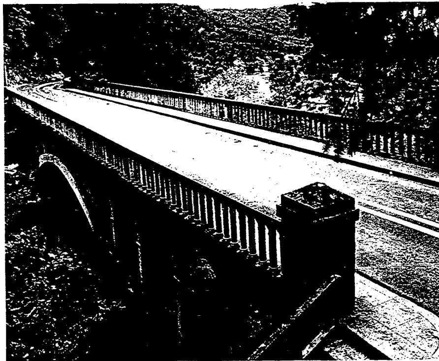
Fig.15c. The new concrete spindles have been installed. This sensitive renovation reused the historic concrete cap railing and stone piers, as they were still in sound condition.
