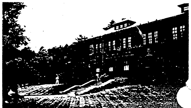
(d.) Hunnewell Visitors Center's entrance following rehabilitation, integrating an accessible path (left), platform, and new steps. Photo: Charles Birnbaum.
