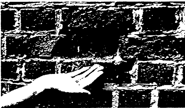
Spalling Brick. This soft, early 19th-century brick was sandblasted in the 1960s; consequently, severe spalling has resulted. Some bricks have almost totally disintegrated, and will eventually have to be replaced. (Robert S. Gamble)
