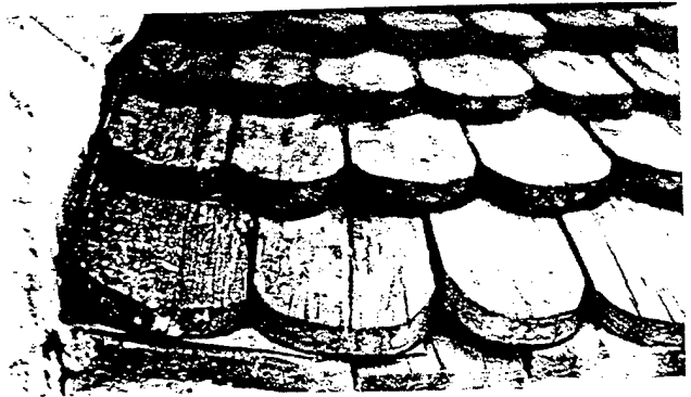
Replacement of particular historic details is important to the individual historic character of a roof, such as the treatment at the eaves of this rounded butt wood shingle roof. Also note that the surface of the roof was carefully sloped to drain water away from the side of the dormer. In the restoration, this function was augmented with the addition of carefully concealed modern metal flashing. (Mount Vernon, Virginia)
