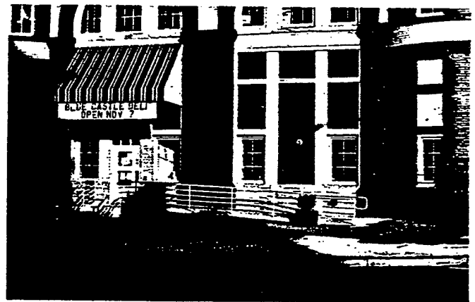
Figure 11. Simple, contemporary railings that extend beyond the ramp slope make this ramp compatible with the industrial character of this building. Photo: Thomas Jester.
