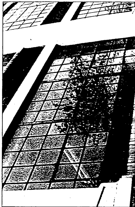
The steel pivot windows in this historic manufacturing building were replaced with new windows which matched the multi-lighted originals.
