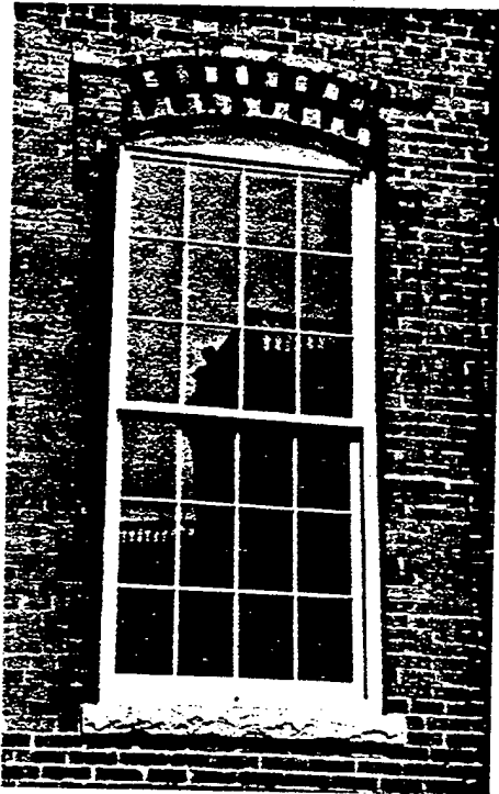
Figure 8. Replacement window sash after installation. Photo: Charles Parrott
