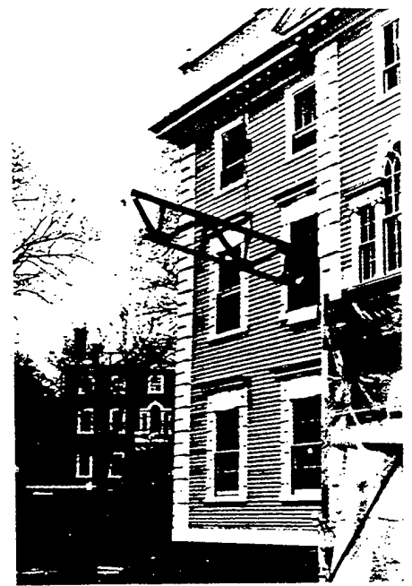
Figure 2. Because of the fire risks, open flame cutting and welding deserves careful attention both in the preparation of specifications and during the work. As much welding as possible should be done off site. For example, at the Nightingale-Brown House, several large trusses were assembled off site, then carefully hoisted through a window for installation. Photo: Irving B. Haynes and Associates.
