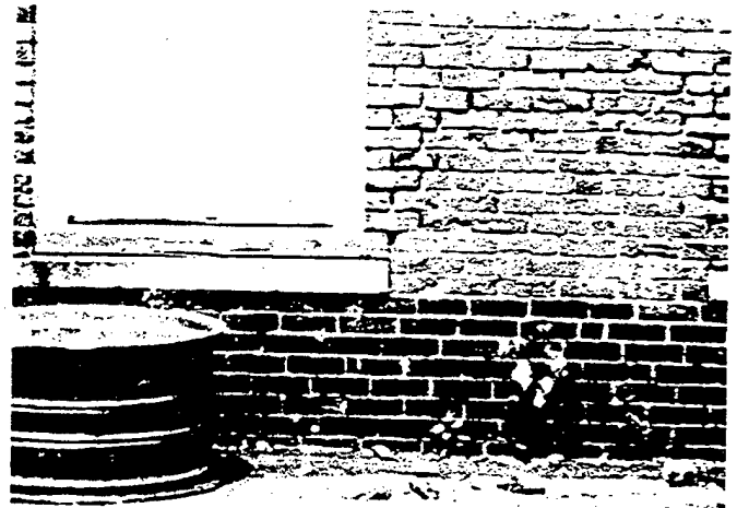
Figure 1. All buildings and building materials are in a constant process of deterioration, such as the brick masonry seen here. Through repointing, the deteriorated mortar joints which might otherwise lead to serious damage, can be renewed and thus preserve the historic character and integrity of the brickwork. Photo: Baird M. Smith.
