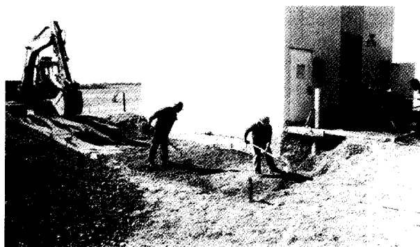
Figure 6. Excavation of foundation.
