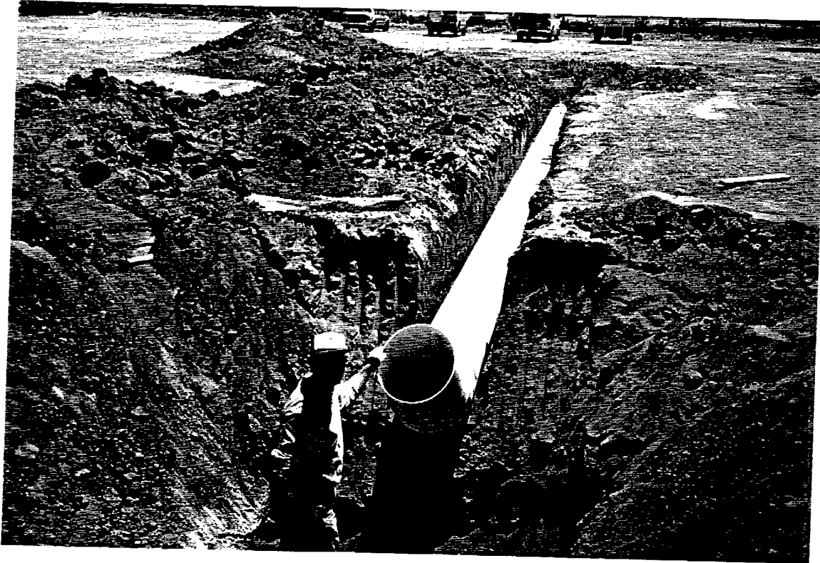
Figure 10: A picture showing the construction of the buried-pipe test facility.
