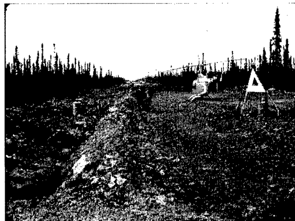
Figure 3. Peat plateau site 84-5B, in the spring after construction (28/04/84). Travel side is on the right.
