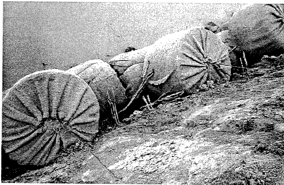
Figure 10. Vegetation in the form of dormant willow posts (discussed later) placed landward of rock and hay bale toe
