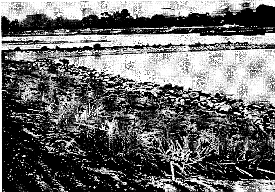
Figure 12. System of bioengineering treatments such as geotextile coir mats with planted vegetation on them placed above a rock roll toe and between large rock transverse dikes
