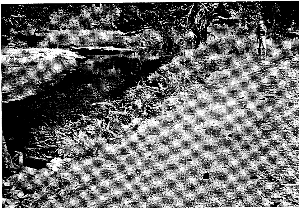
Figure 20. Root wads soon after installation on Upper Truckee River, California, near South Lake Tahoe (Voids within and between root wads are filled with a soil mix and planted with live, vegetative clumps or root pads, such as willow)
