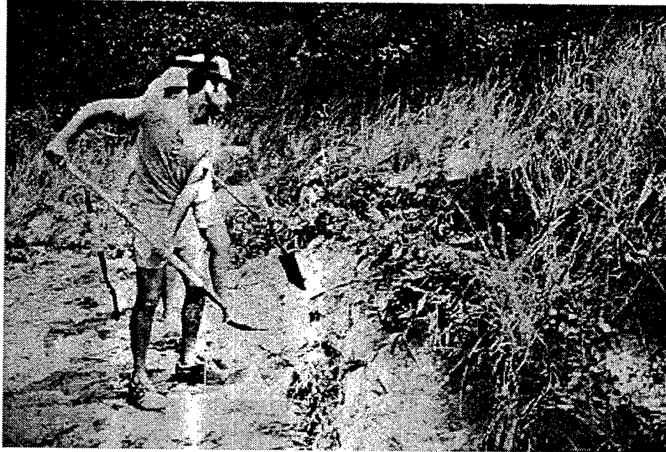
Figure 29. Installed section of brush layering (Note that brush has leaves because of a workshop setting. Normally, brush would be without leaves because of installation during dormant season)
