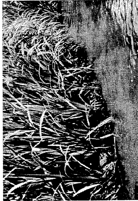
d. Closer view of coir roll a few months after plant establishment
