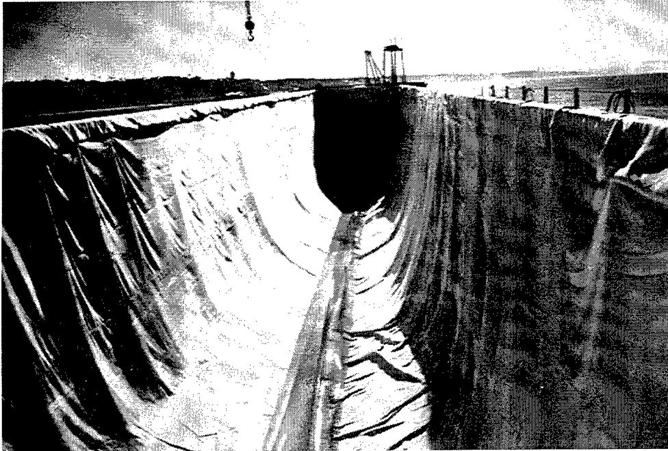
Figure 7. Geotextile liner inside a split-hull scow used in the Marina del Ray contaminated material containerization project
