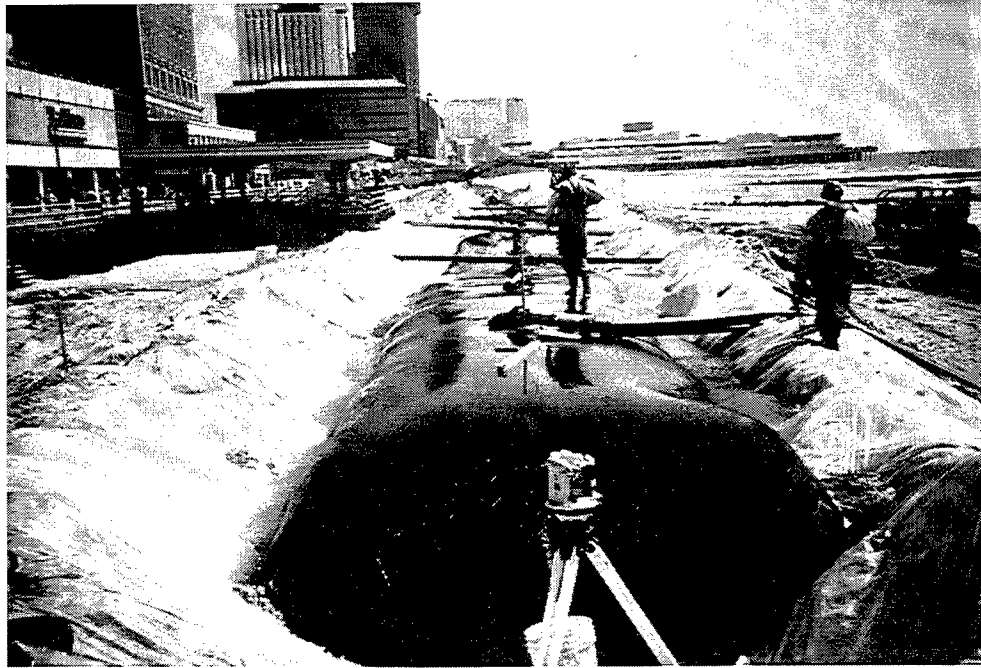
Figure 1. Construction of the geotextile tube in front of the Atlantic City, NJ, boardwalk
