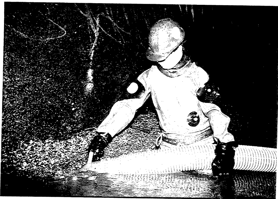
Figure 5. Removal of zebra mussel shell debris by vacuum hose (photographed by Peter Yates)
