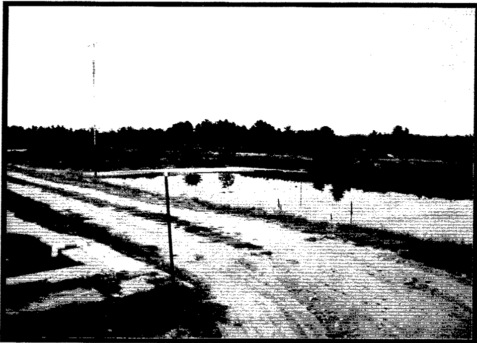
11. AREE 20 - TYPICAL RAPID INFILTRATION BASIN
