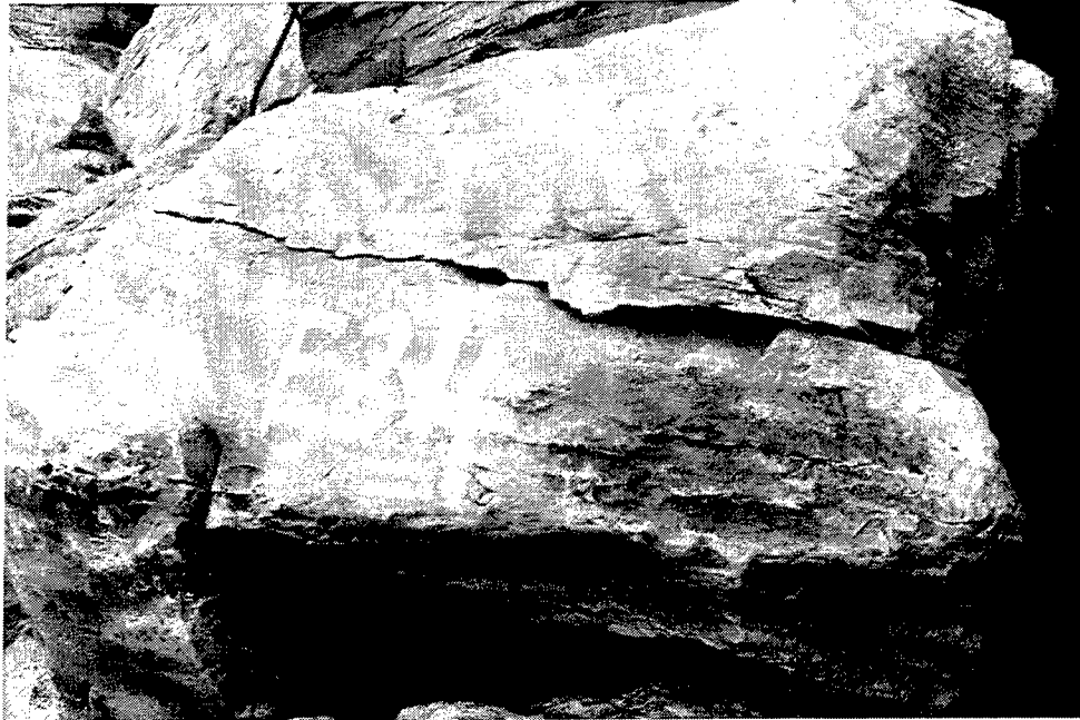
Figure 40. View of broken armor stone on St. Paul Harbor breakwater (station 10+21)
