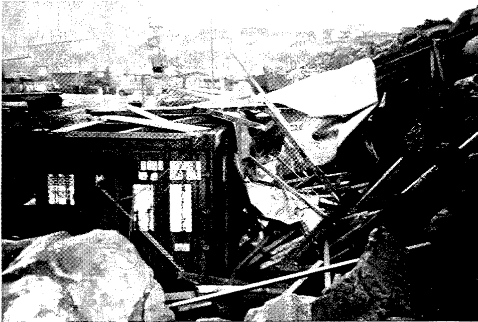
Figure 22. Collapsed apron resulting from 3 November 1994 storm
