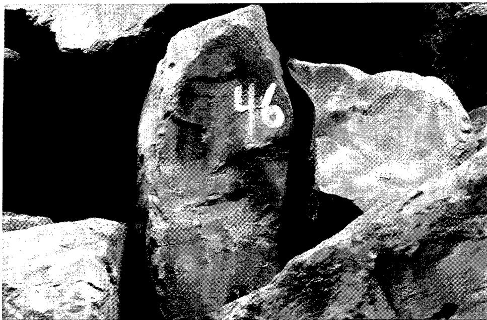
Figure 41. View of broken armor stone on St. Paul Harbor breakwater (station 11+78)
