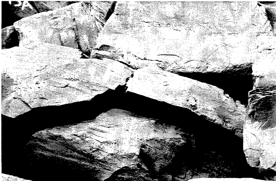
Figure 43. View of broken armor stone on St. Paul Harbor breakwater (station 17+34)
