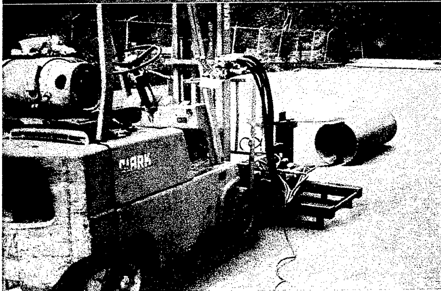
Figure 29- Combined RPPC and HPG Pile Cutting Operation (cont.)
