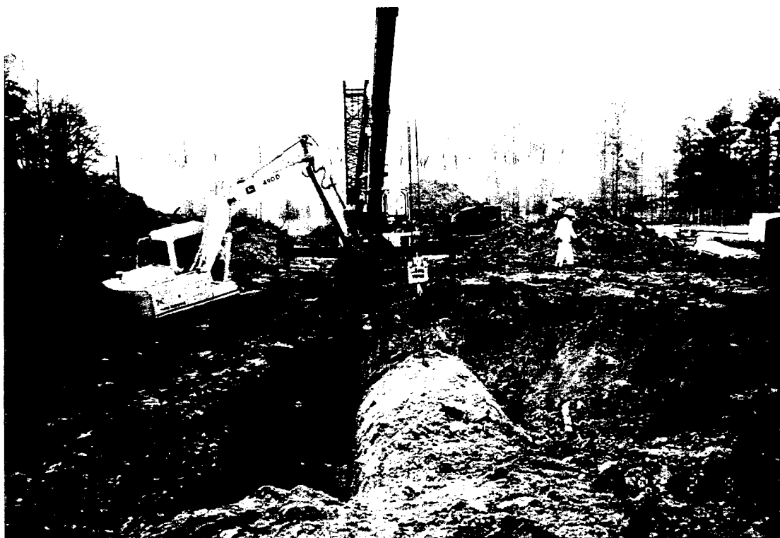
Site 4 - UST No. 4 Removal. View to the North. (Photo Log No. 7; Roll No. 6/Frame No. 3)
