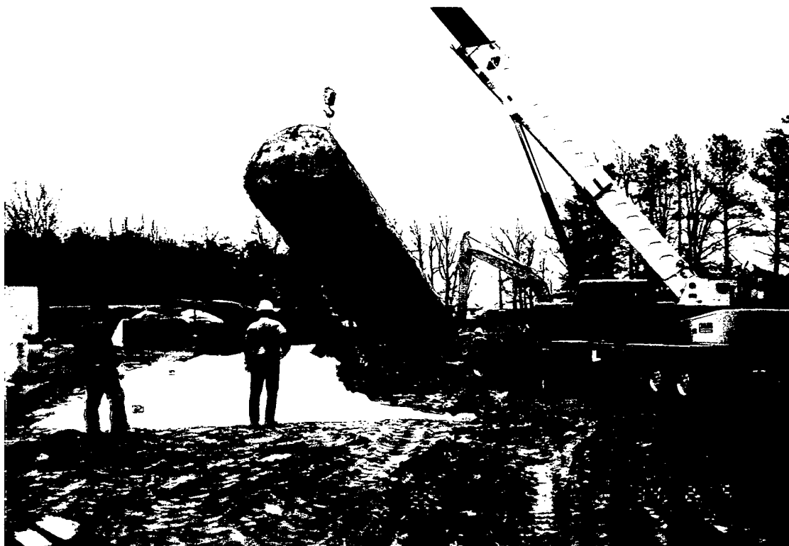
Site 4 - UST No. 4 Removal. View to the South. (Photo Log No. 7; Roll No. 6/Frame No. 20)
