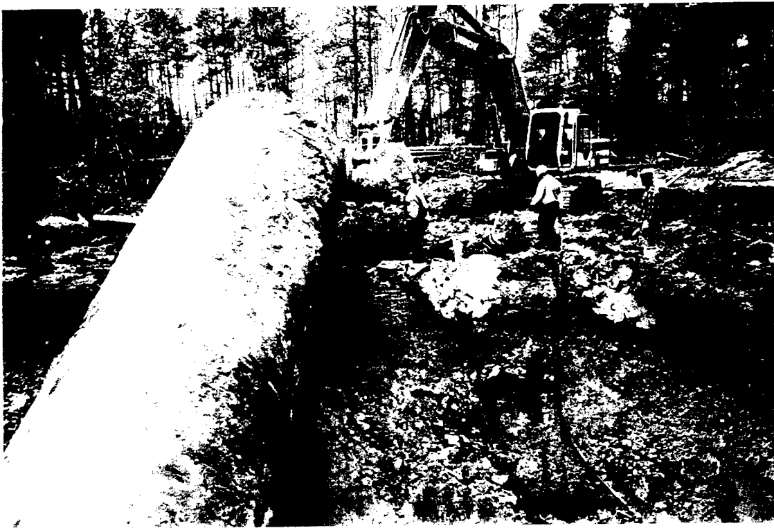
Site 5 - UST No. 11 Removal. View to the West. (Photo Log No. 5; Roll No. 2/Frame No. 27)
