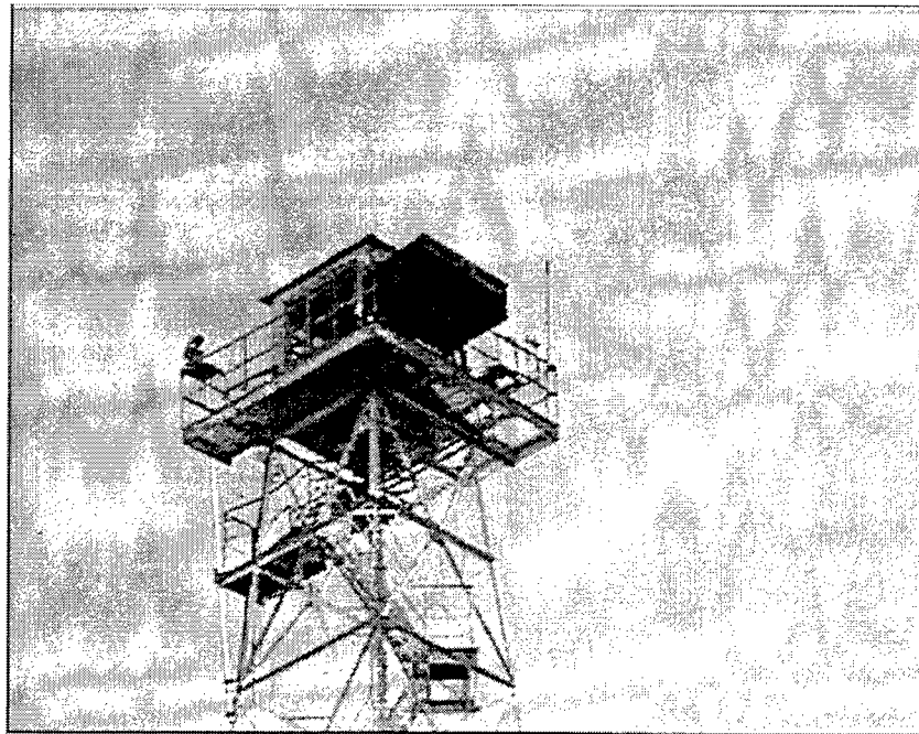
Figure B1. The FRF'S's 42-m-tall observation tower. The photo shows the housing for the fixed-look video cameras(the remote control camera is on the leftmost corner)
