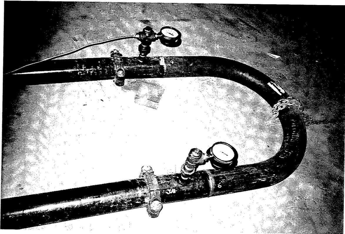
Figure 12. Pressure gauges installed at the bend on pipeline
