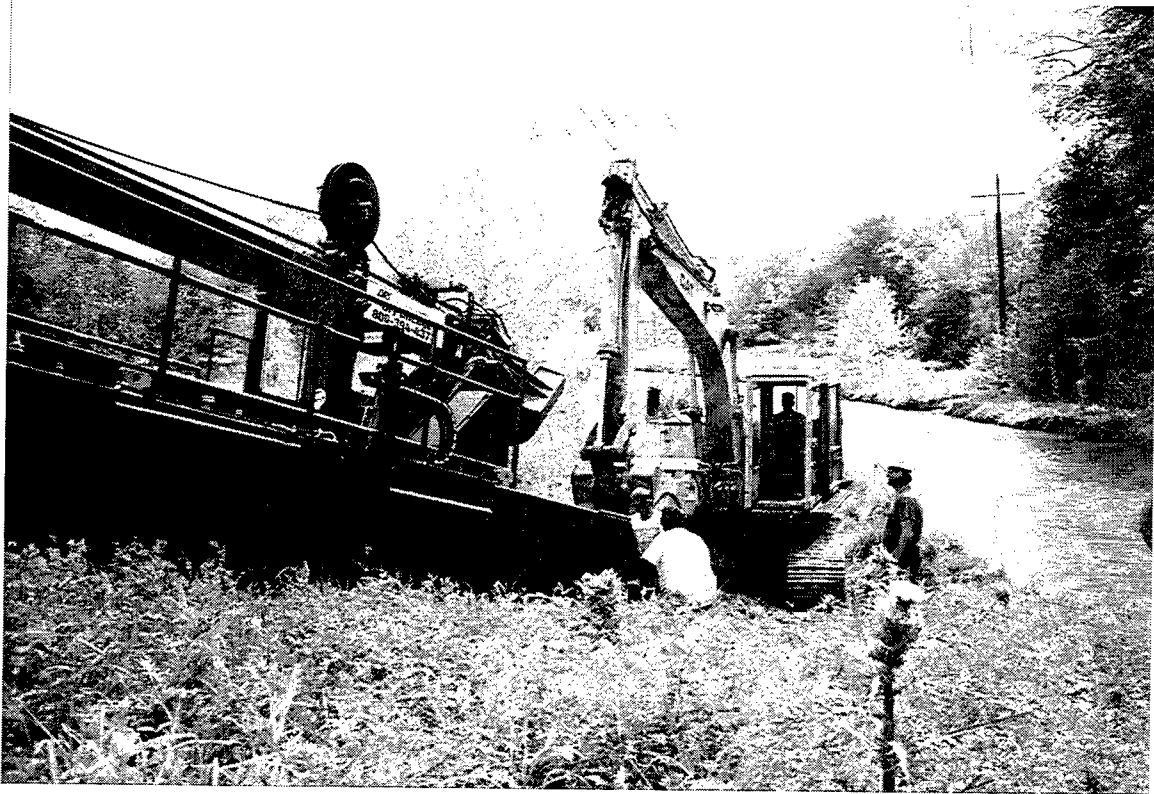
Figure 19. Transportation of Dry DREdge™ towards lake
