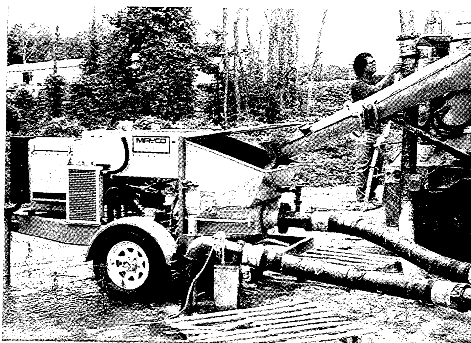
Figure 9. View of hopper attached to pump for temporary storage of sediment
