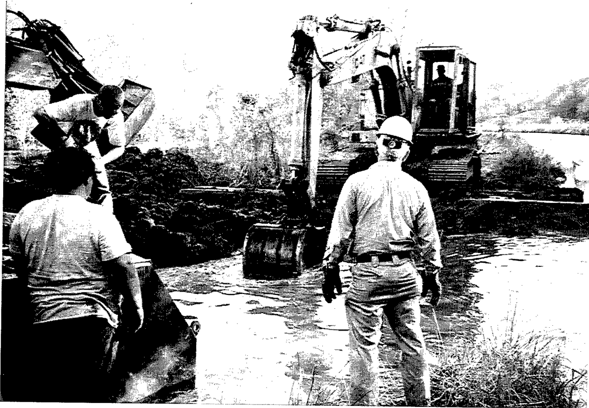
Figure 21. Channel being dredged for launching
