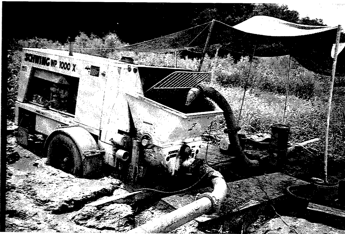
Figure 29. Booster pump halfway on the pipeline
