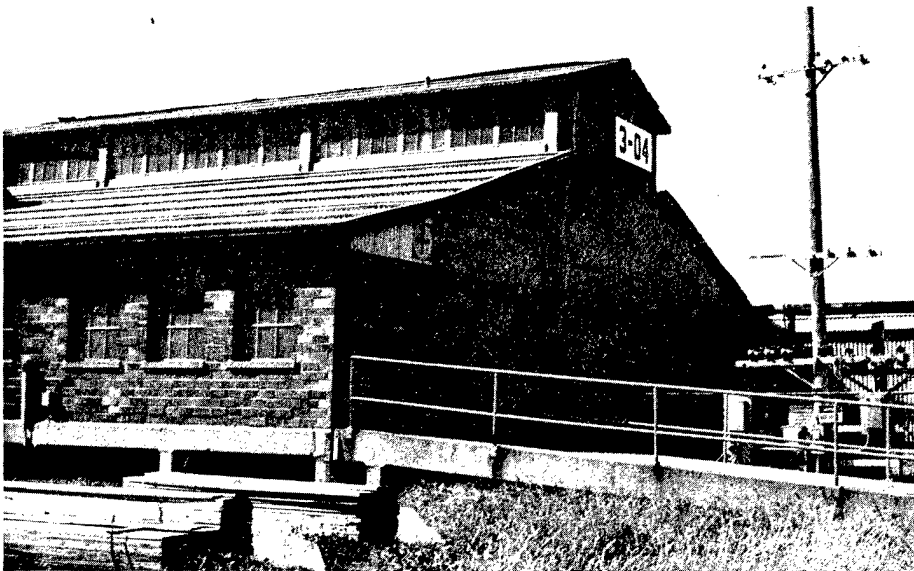
Typical Line Building Construction.
