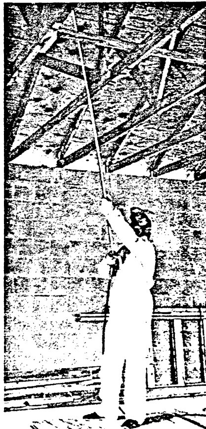
Spray-applied interior radiant barrier is installed on the underside of the roof deck.
