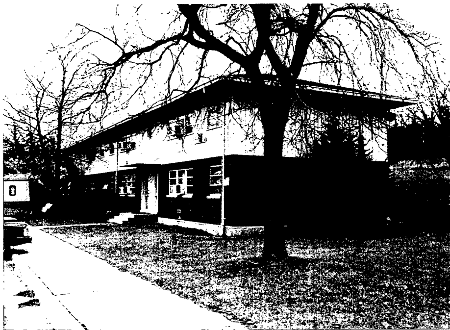
PHOTOGRAPH NO. 9 - BUILDING 621 SOUTH AND EAST ELEVATION
