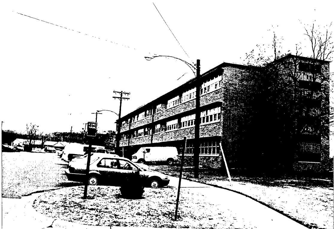
PHOTOGRAPH NO. 6 - BUILDING 610 SOUTH AND WEST ELEVATIONS
