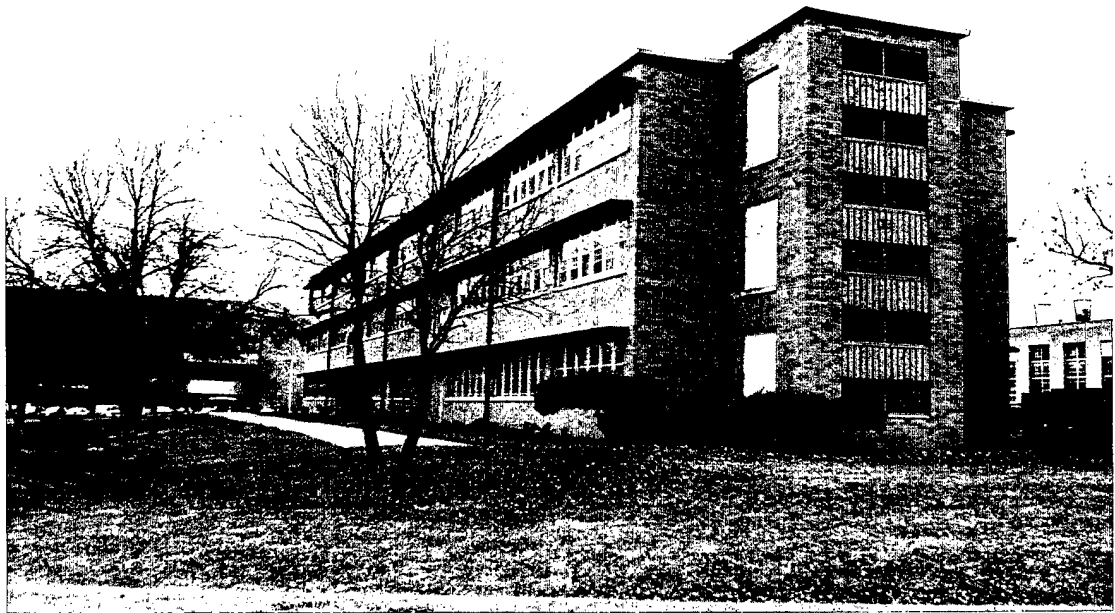
PHOTOGRAPH NO. 5 - BUILDING 610 NORTH AND EAST ELEVATIONS
