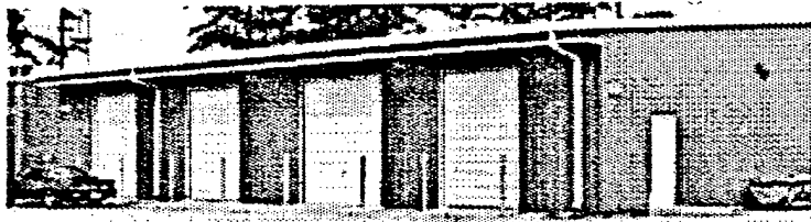
Left: The exterior of building 4183
