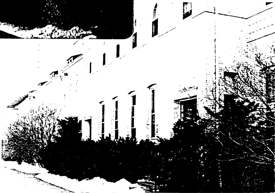
Figure 19 Bldg. No. 48 General Administration category historical Faces parade ground
