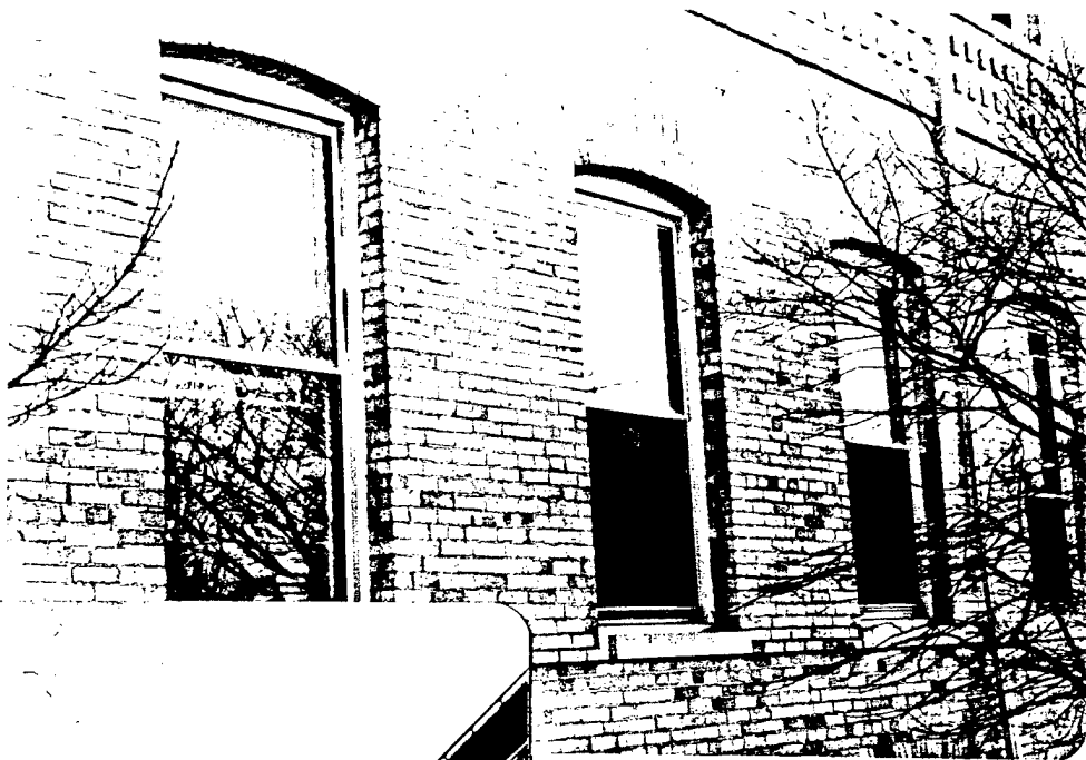
Bldg. No. 48 Administration category - historical recent storm window and window caulking modifications
