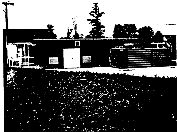
In many large installations (as at left), blender, controls, air compressors are inside a building.
