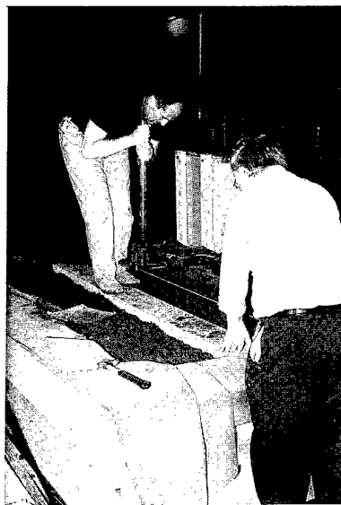
b. Tamping planks into trench.
