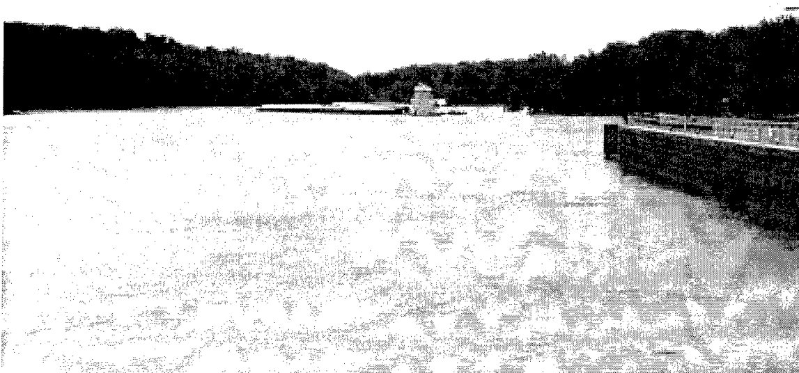
Photo 4. Path of downbound tow entering channel, looking downstream
