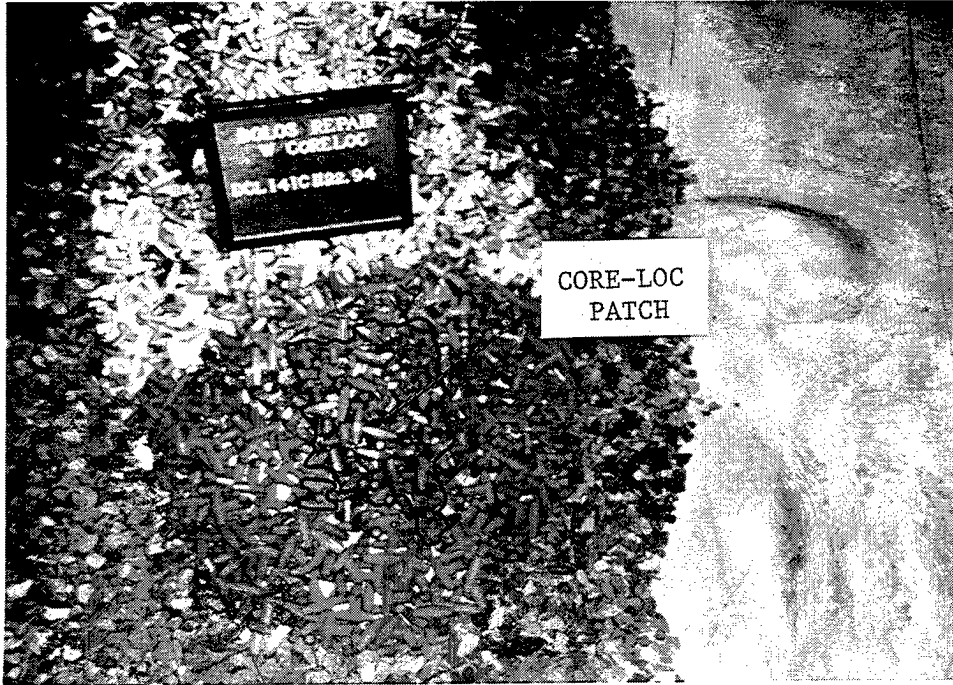
Photo A3. TS1, Core-Loc repair of dolosse armor
