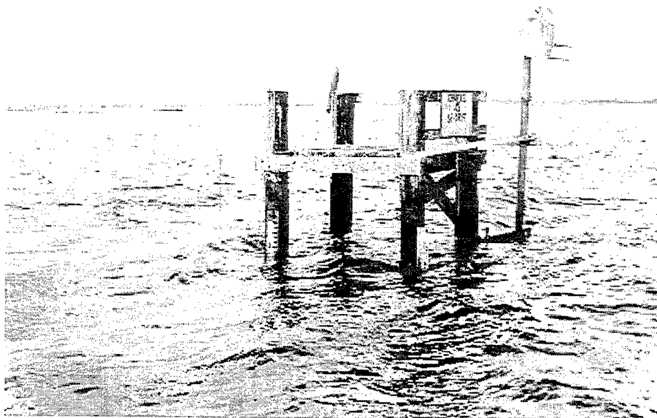
Figure 8. Tide staff mounted on survey table at Channel to Victoria (see Staff 8, Chart G, Appendix B). A dredging contractor's staff is mounted on the third pile from left
