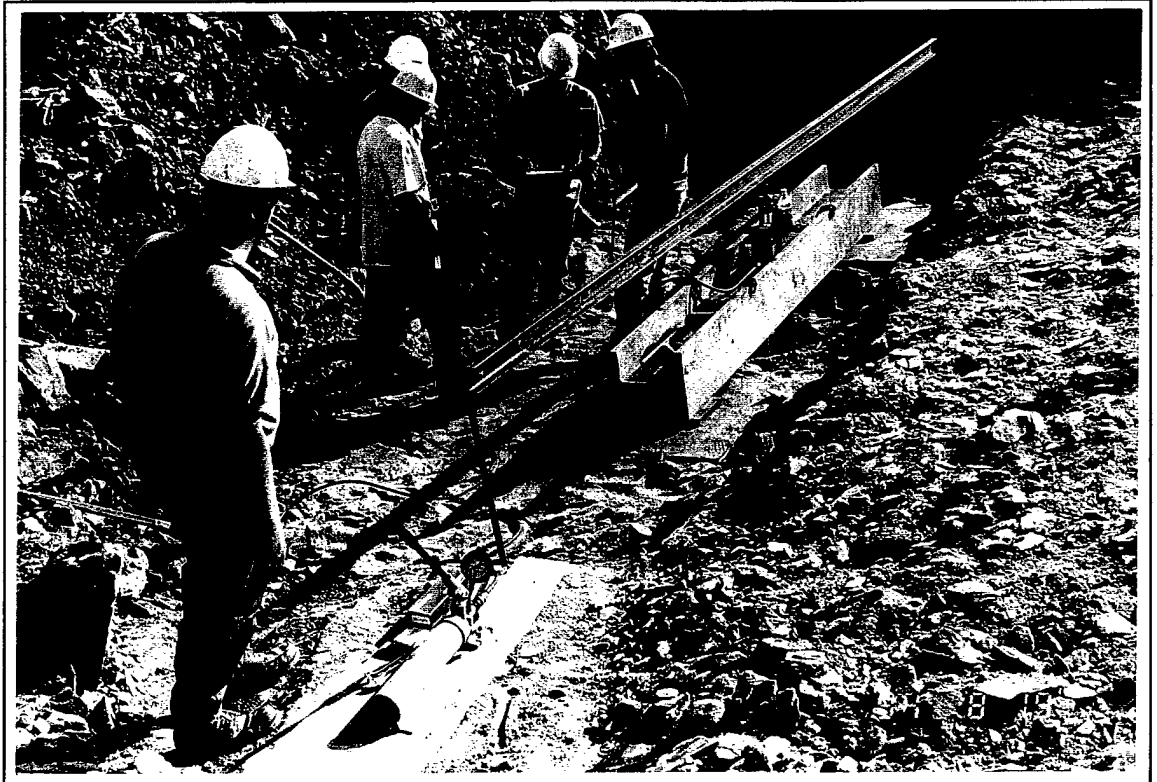
Photo 15. Setup for the anchor pullout test.
