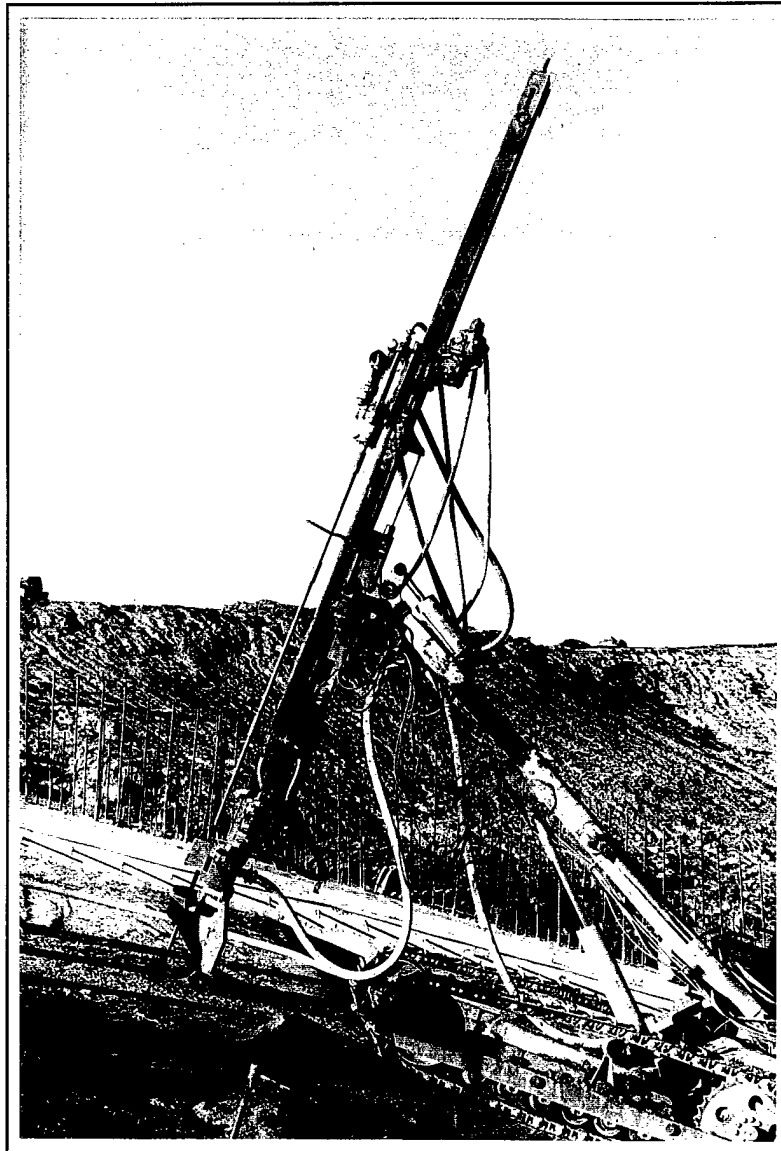
Photo 14. Drilling anchor holes.
