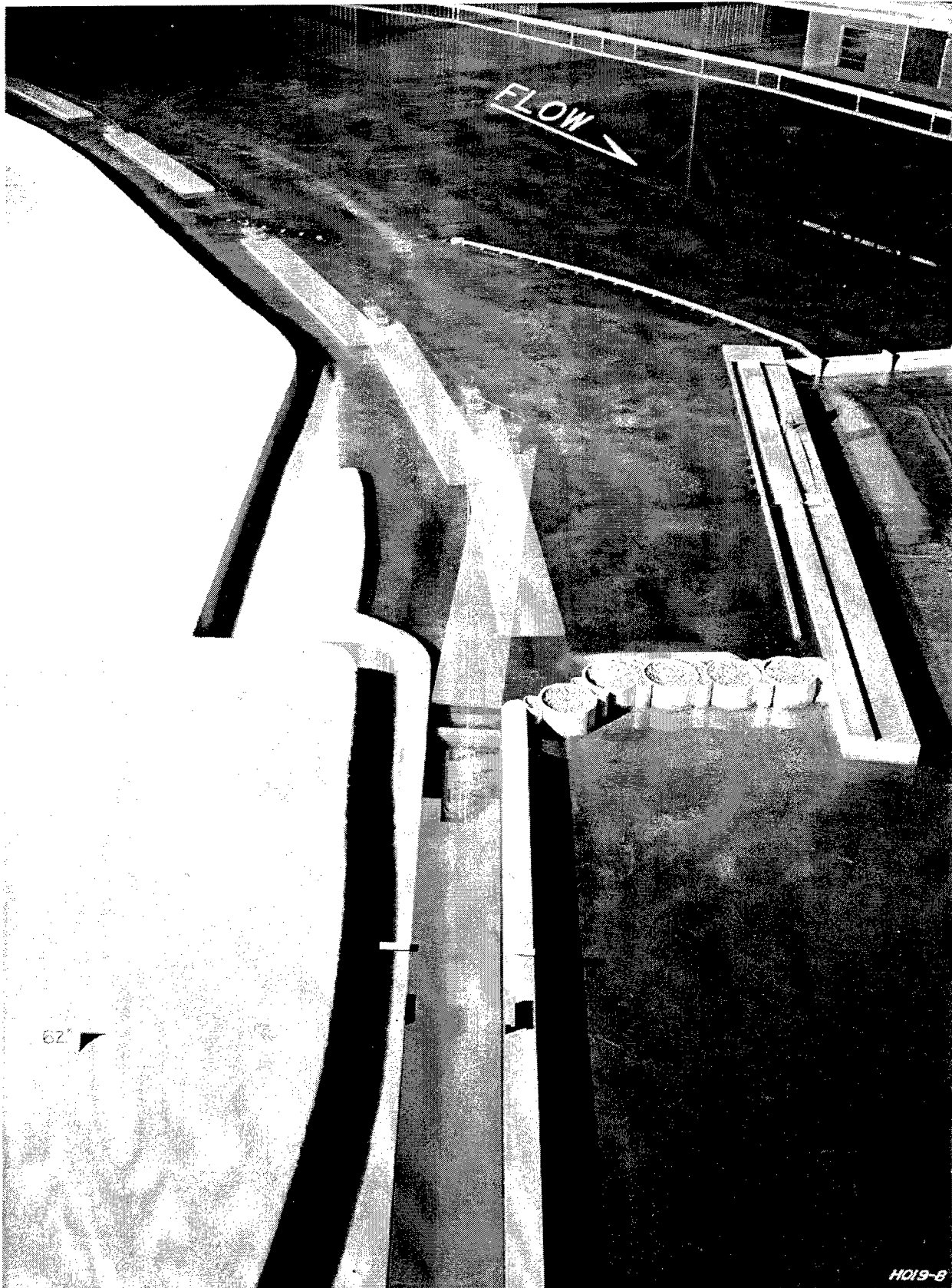
Photo 3. Base Test, total riverflow = 62,000 cfs, powerhouse discharge = 62,000 cfs. Looking upstream, showing the path of downbound tow approaching and entering the lock (note maneuvering required to enter lock)
