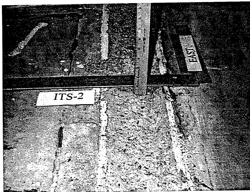
Figure 76. Close-up view of failure plane under east wall of ITS-2.
