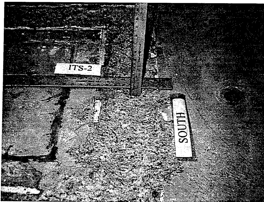
Figure 78. Close-up view of failure plane under south wall of ITS-2.
