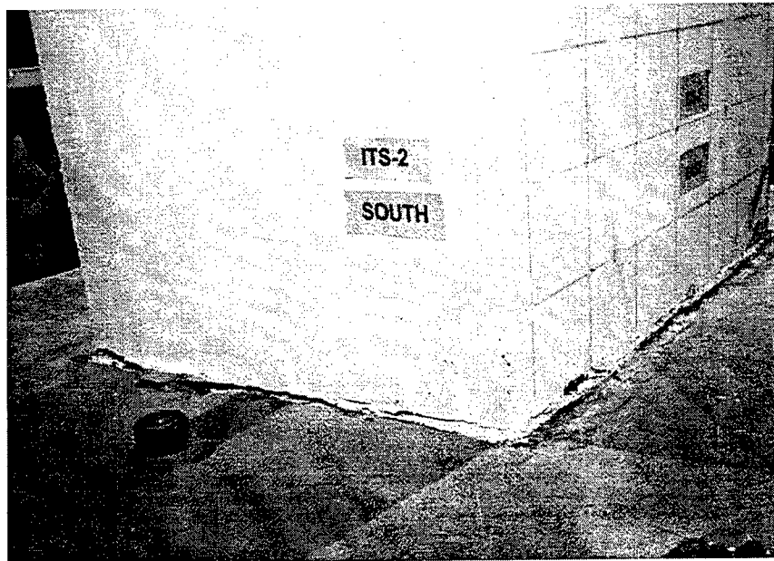
Figure 71. ITS-2 view of south and east walls, imposed top deflection of 2 in. east.
