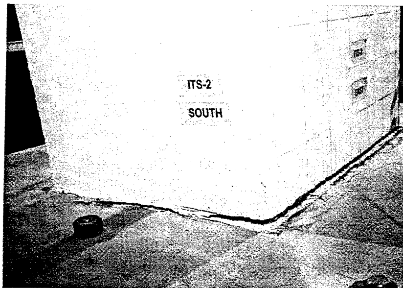
Figure 70. ITS-2 view of south and east walls, imposed top deflection of 2 in. west.
