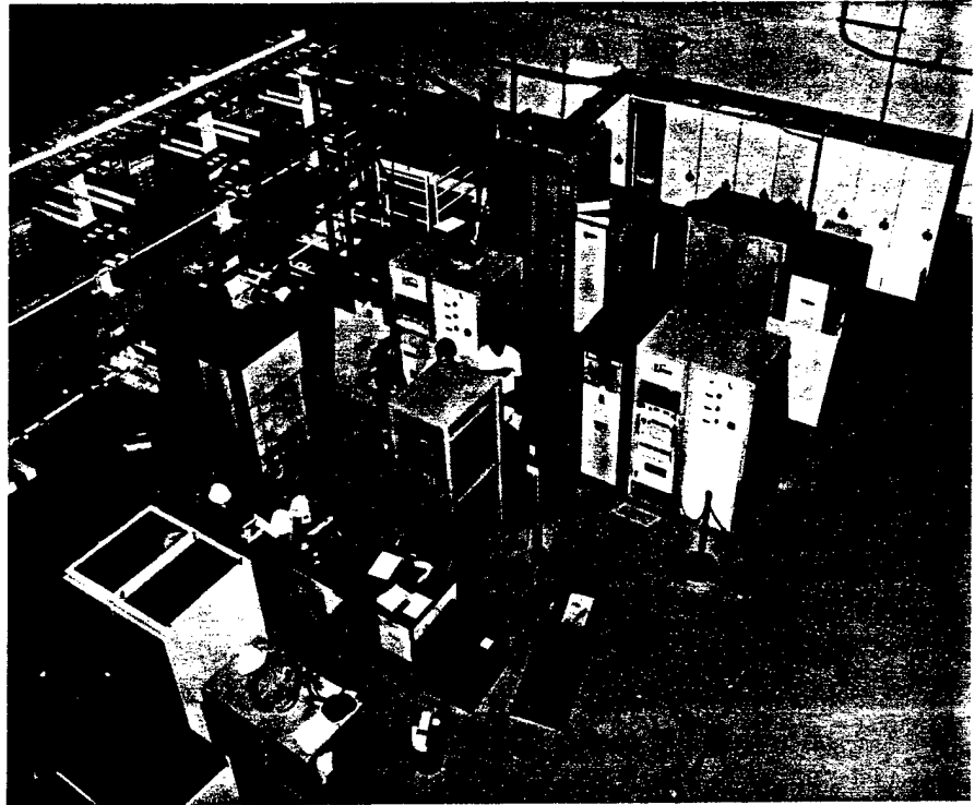
Figure 5.18. View of initial installation of tetrode amplifiers for GTA.
