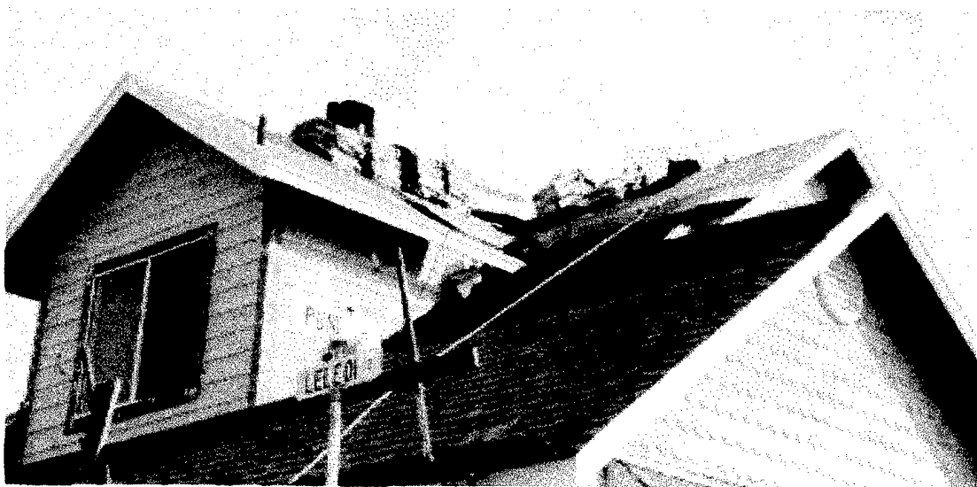
Figure B.6: New construction, Ewa Beach; PR20 Eave Catchguard system and Trus-T PFAS variant, corner view
