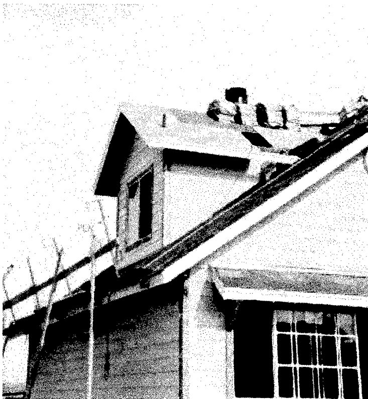
Figure B.5: New construction, Ewa Beach; PR20 Eave Catchguard system and Trus-T PFAS variant, end view
