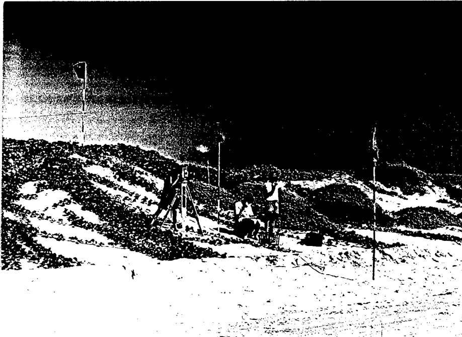
Figure 9. Survey crew operating electronic total station.
