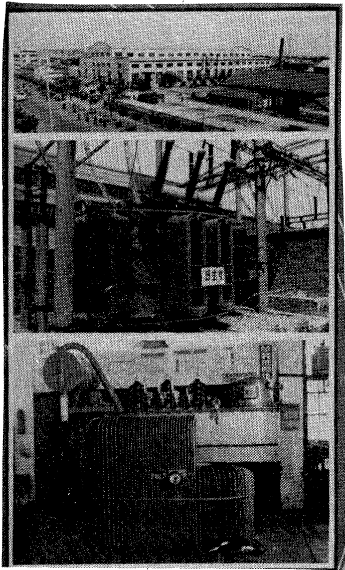
Fig. 22 Photograph of the Lianyungang Transformer Plant in Jiangsu Province. Products include large, medium, and small electric transformers, transformers for carrier voltage regulators, electric furnaces, rectifiers, low tension strong electric current salt-bath furnaces and mines. The capacity of the transformers ranges from 10KVA to 31500KVA, and the class of voltage from 110KV down. [Source: Hong Kong ZHONGGUO JIXIE [CHINA MACHINERY] in Chinese and English No 4, 1983, back cover]
