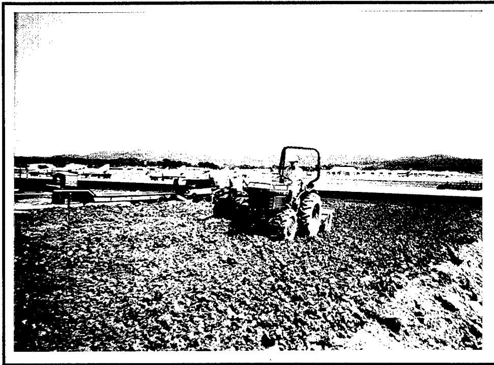
Photo No. 9: Tilling of soil in a bio-cell.
