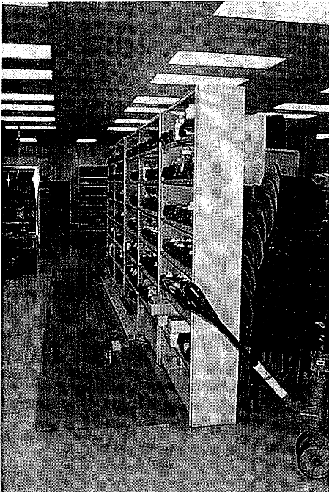
Figure 35. Unanchored tall narrow shelves.
