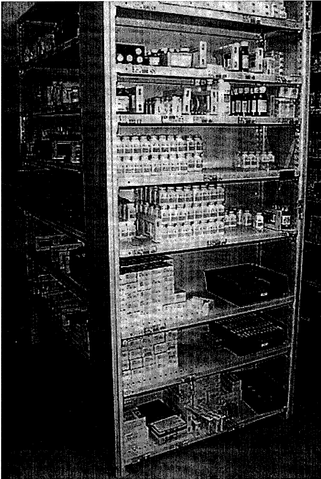
Figure 34. Unanchored tall narrow shelves that may be secured in their present configuration.
