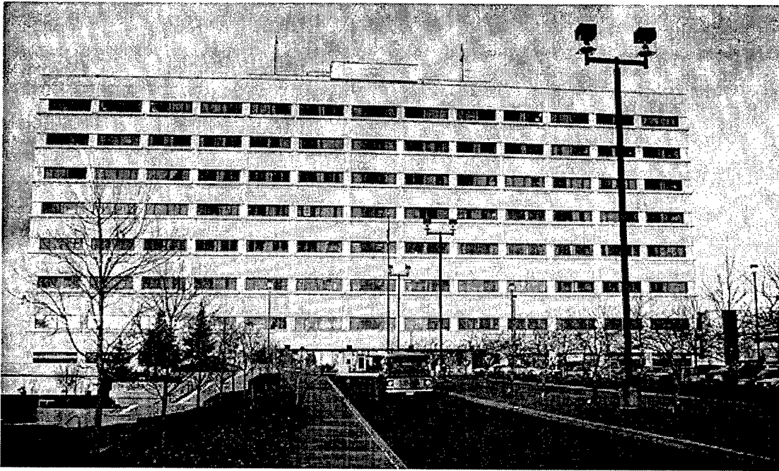
Figure 1. East side of the Nursing Tower at MAMC.
