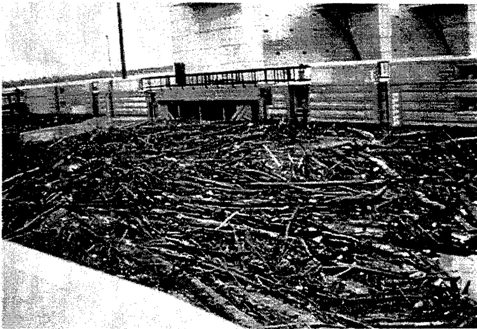
Typical log jam, Lock and Dam Operation
