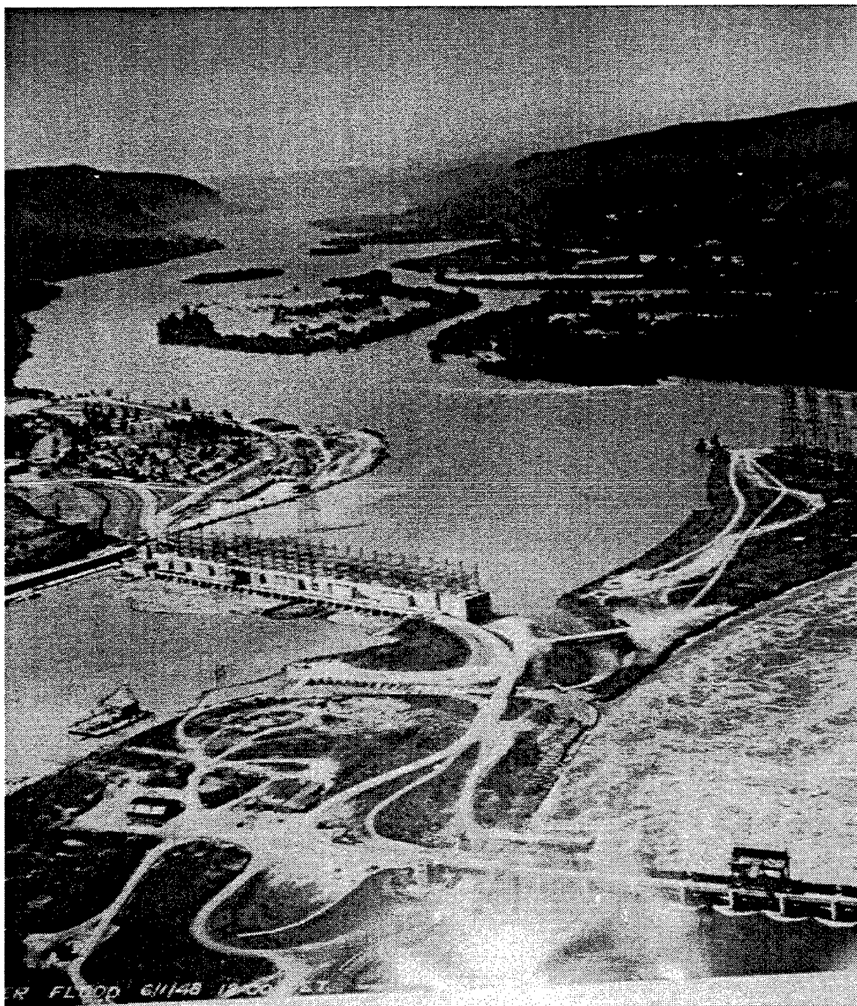
Bonneville Powerhouse No. 1 with debris jam in 1948
