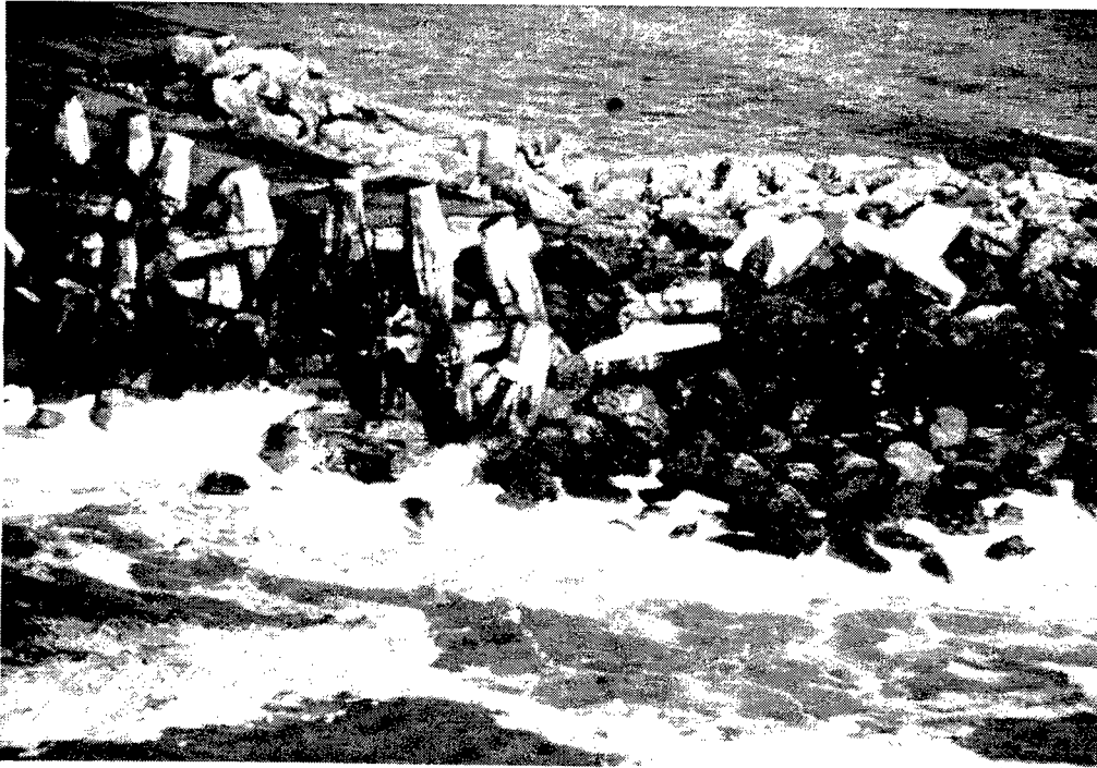
Figure 1. 1982 breakwater damage at Crescent City, CA. Note the broken dolos and scattered armor stone
