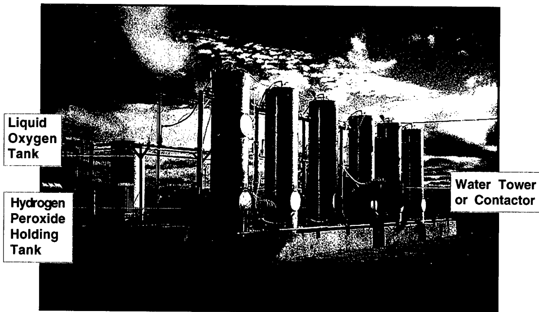
Figure 2. The Peroxone treatment plant was comprised of six water towers, oxygen tank, ozone generator (not seen), three GAC filters (behind water towers), and holding tanks.
