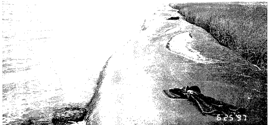
Figure 2. Geotextile tube tears due to ultraviolet sunlight damage
