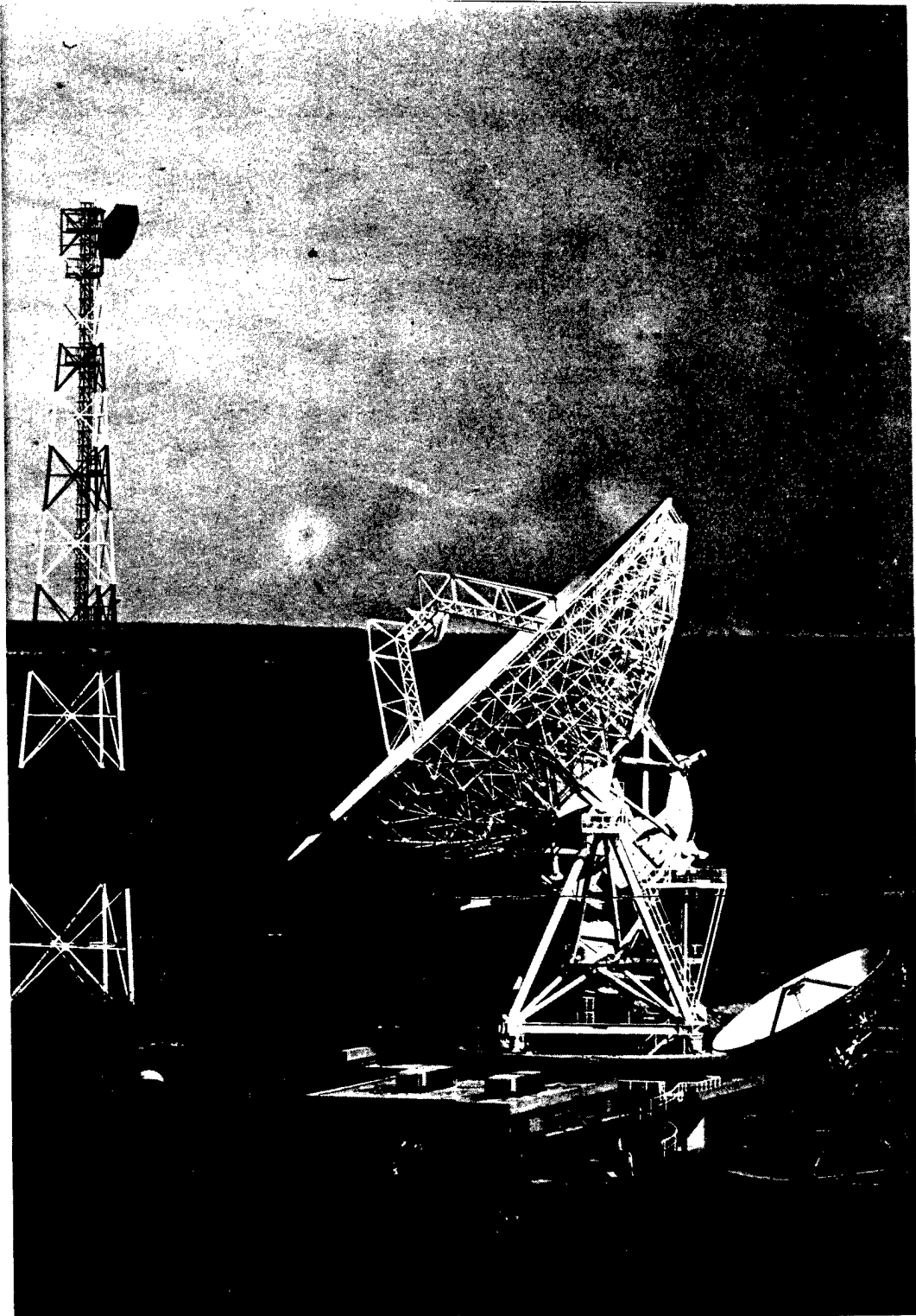
The international satellite earth station at Karma. It will provide telephone and television links throughout Nigeria and with the entire world.
