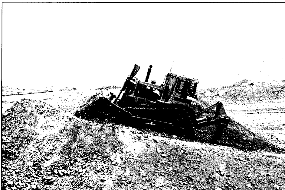
Figure 1. Dozer operation with the automated system.
