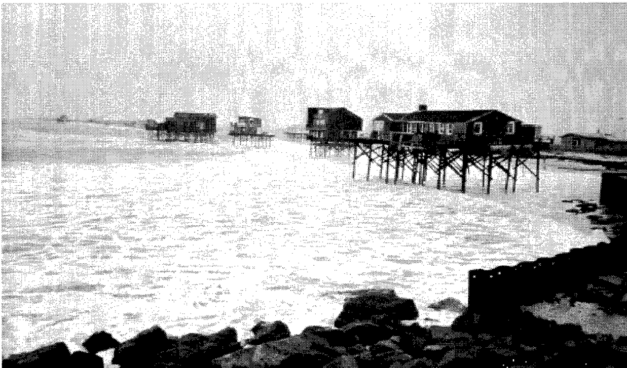
Erosion downdrift of groin field, Westhampton Beach, Long Island, NY.
