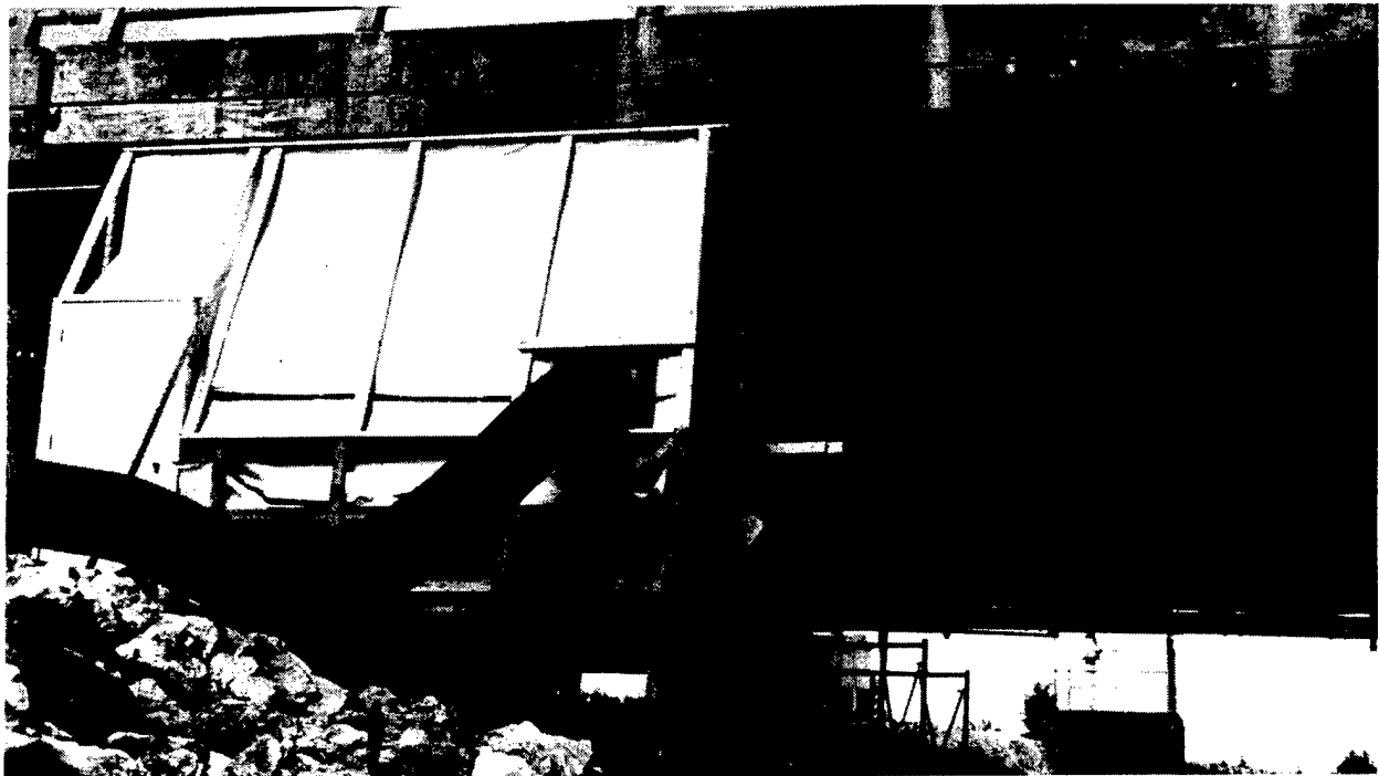
Figure C.6. Containment structure built for the demonstration.
