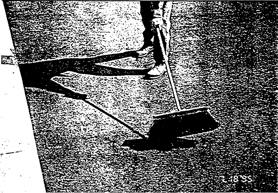
Figure 55. Finished bridge after floodcoating
