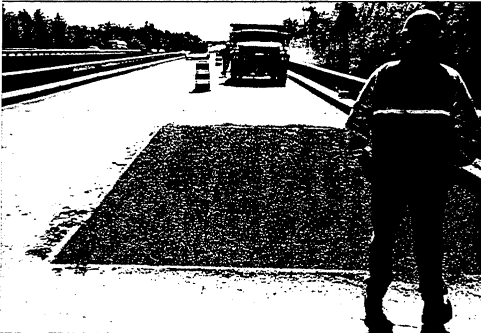
Figure 68. Finished Category-II overlay
