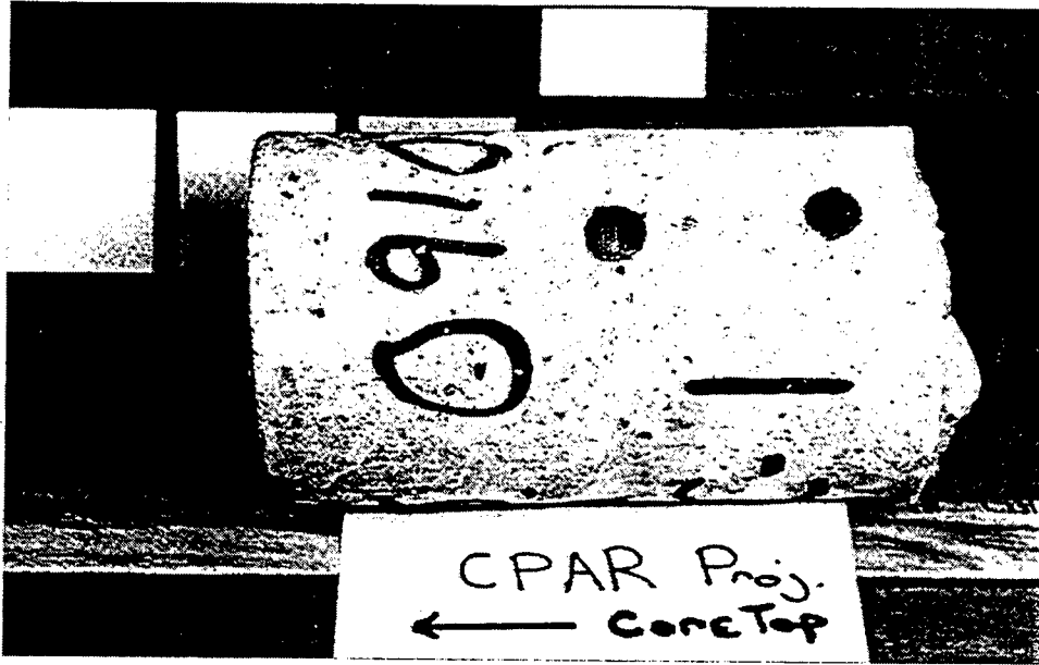
Figure J1. Core Sample No. S05-09101-C-1. Profile view of 4-in.-diam bridge deck core showing overall size, condition, and presence of steel reinforcement (two circular objects imbedded in the concrete)
